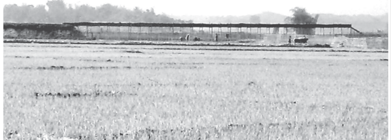
Freshwater from the Kalapanzin Creek is supplied to summer paddy fields through a large aerial gutter.
