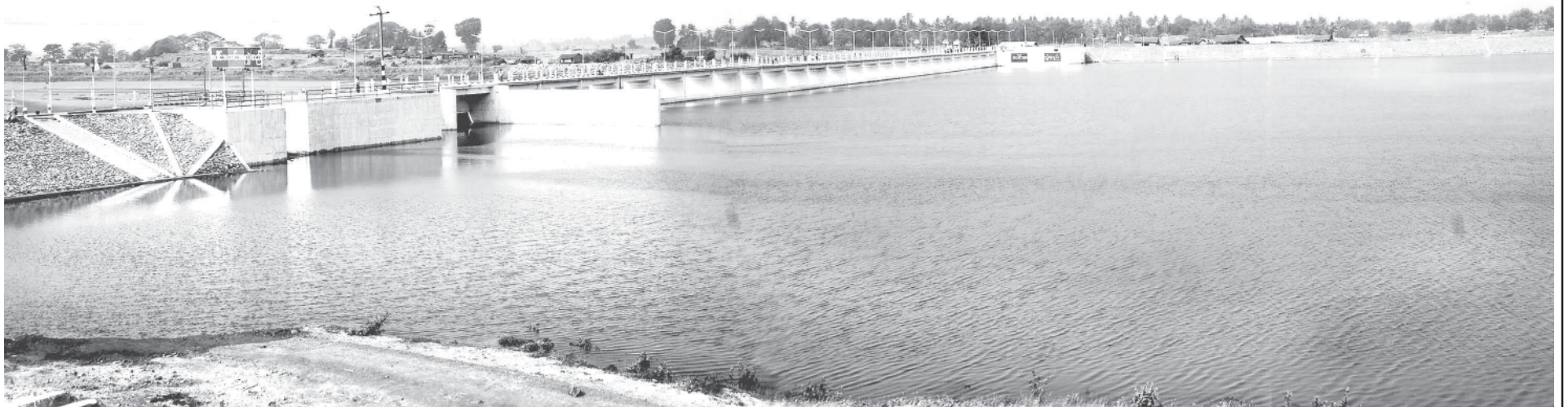
Paunglaung Diversion Weir built near Thitseintpin Village of Nay Pyi Taw Pyinmana Township stores water to be supplied to 35,000 acres of farmlands.
