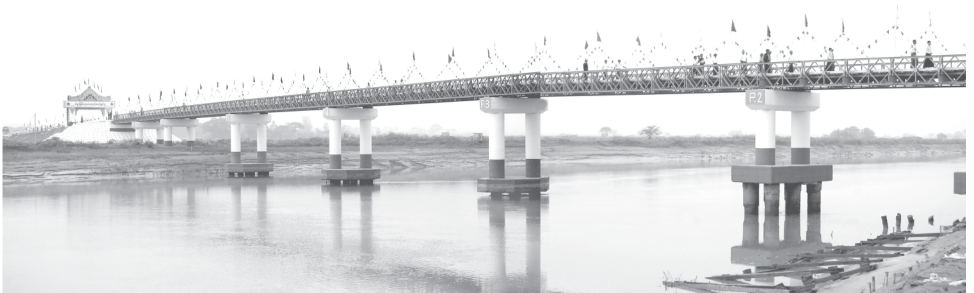
Newly built Bago River Bridge (Kawa).—MNA
