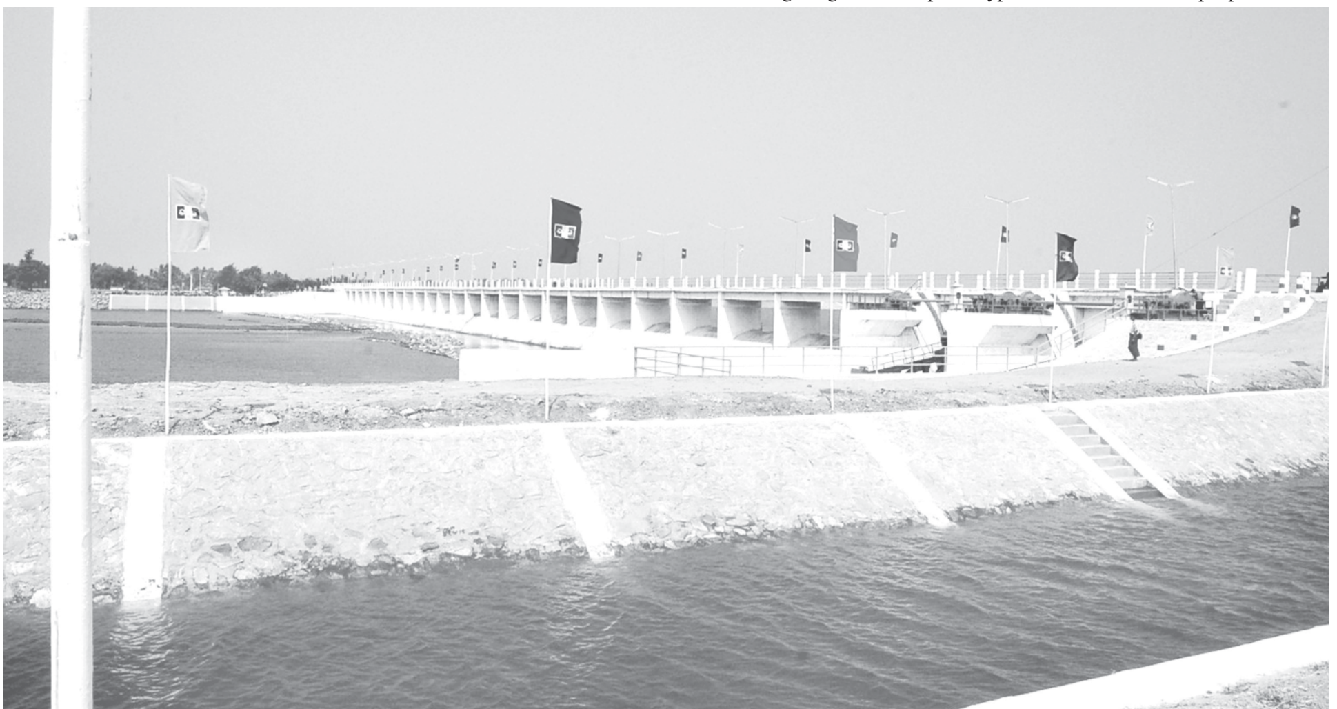
Paunglaung Diversion Weir in Nay Pyi Taw Pyinmana Township.—MNA
