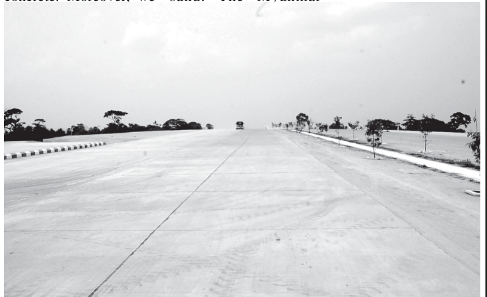
Two Way/Two Lane Concrete section near Myochaung Village on Yangon-Nay Pyi Taw Road.
