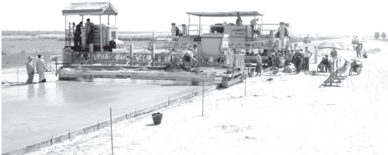
Workers pave concrete on Yangon-Nay Pyi Taw Road Section.
