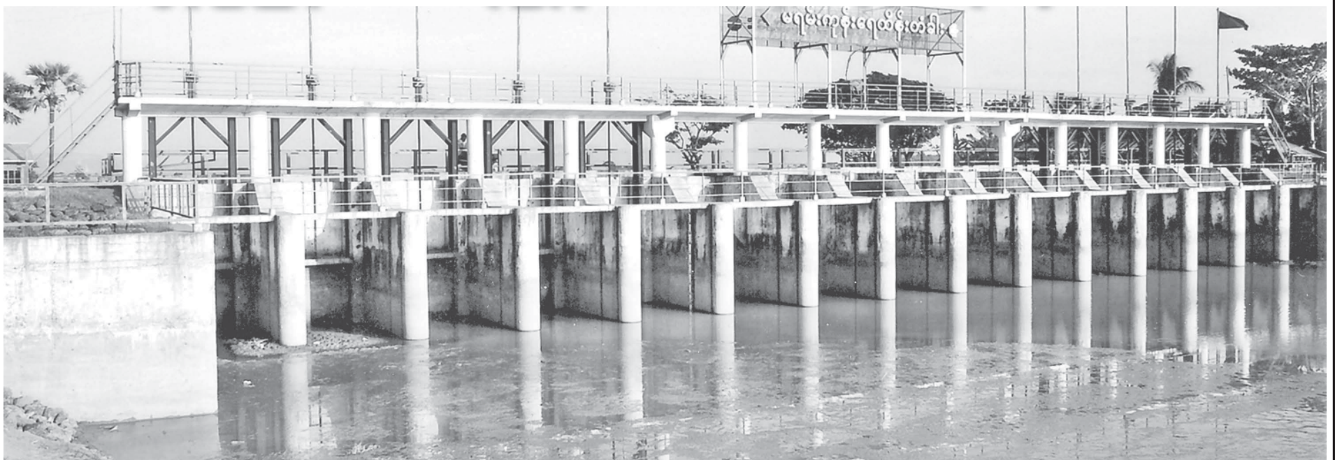
Mayangon Sluice Gate near Mayangon Village, Thaton Township, Mon State.
