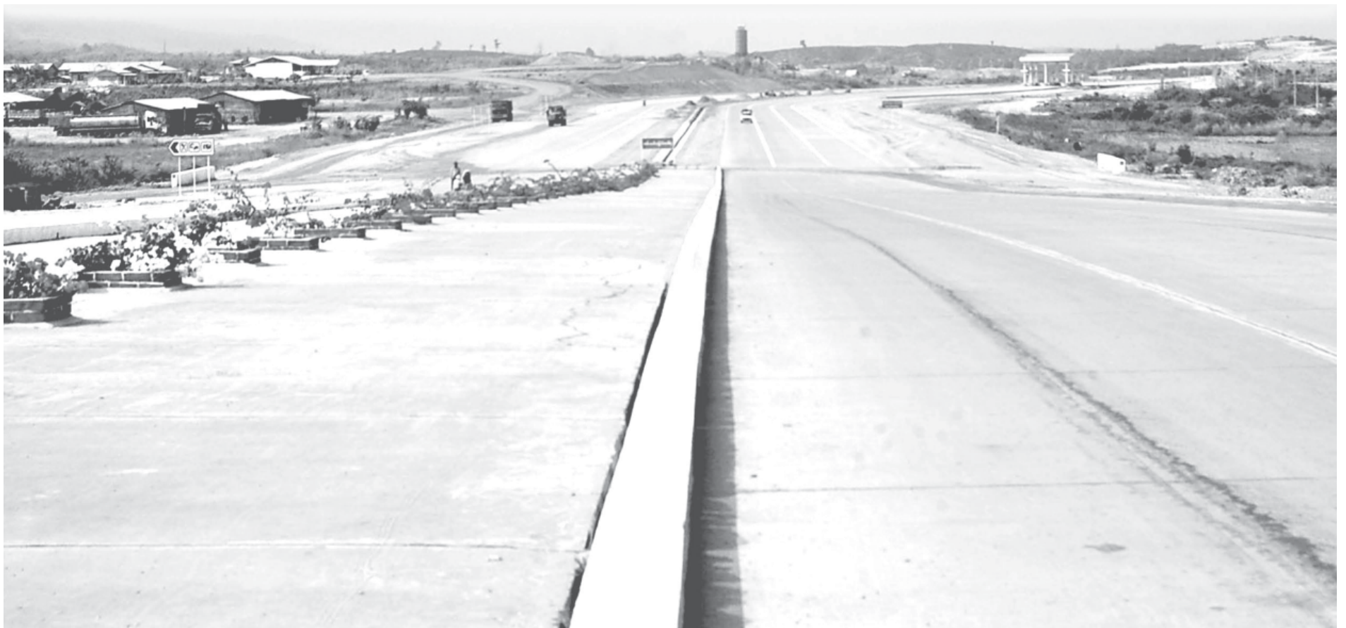
Photo shows progress in constructing the two-way / two-lane concrete road of Yangon-Nay Pyi Taw Road section near Pyu.
