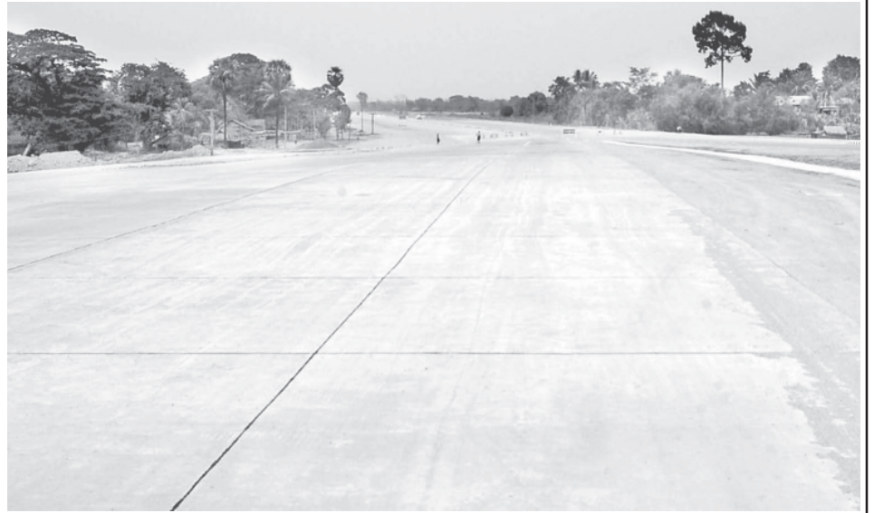
A two-way / two-lane concreted road under construction of Yangon-Nay Pyi Taw road section.
