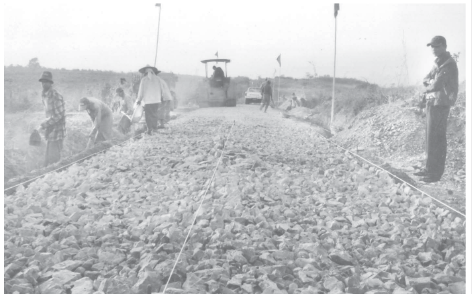
Gravel being placed on Pyinsar-Pauktaw inter-village road.
