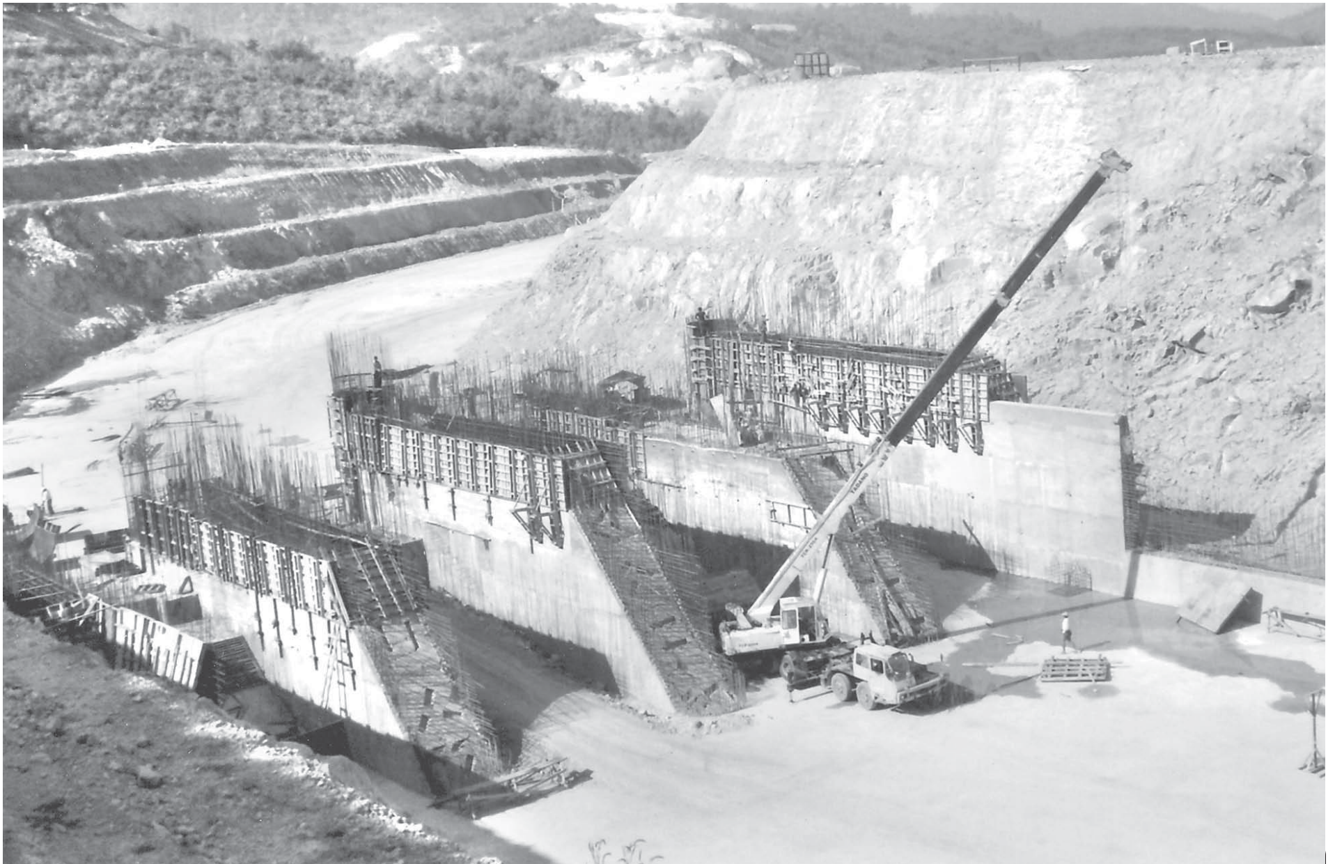
The three-gate spillway of Shwegyin Hydropower Project is under construction.
