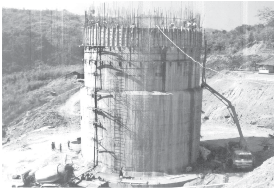
Surge drum is being built at Kunchaung Hydropower Plant.
