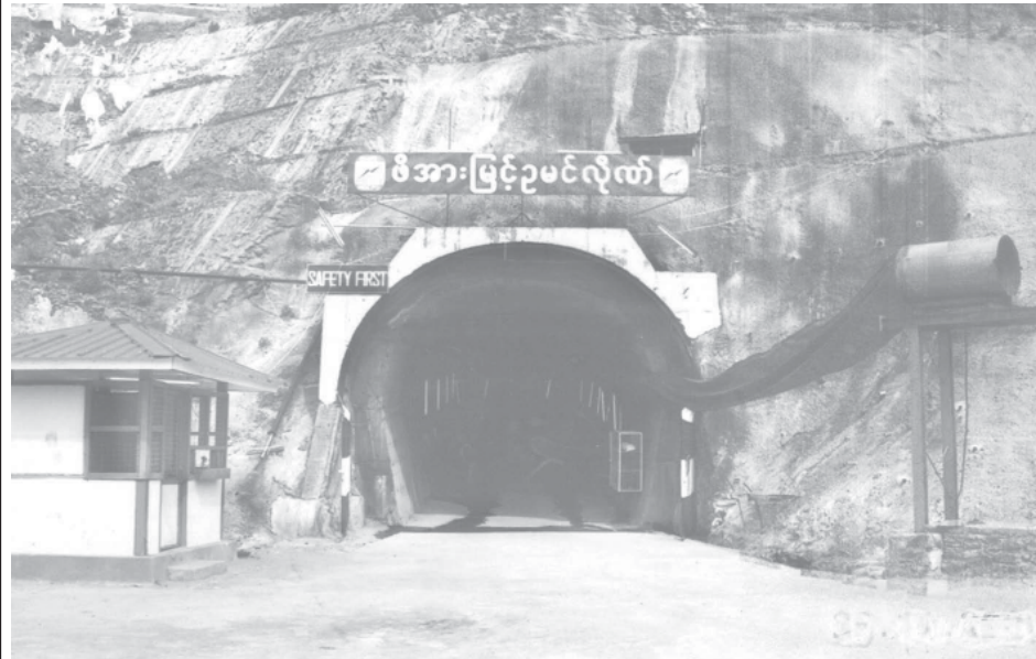
Photo shows penstock tunnel of Kunchaung Hydropower Project.
