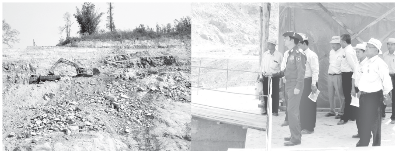
Minister for Electric Power No. 1 Col Zaw Min inspects progress of Nancho Hydropower Project.—EP NO. 1
