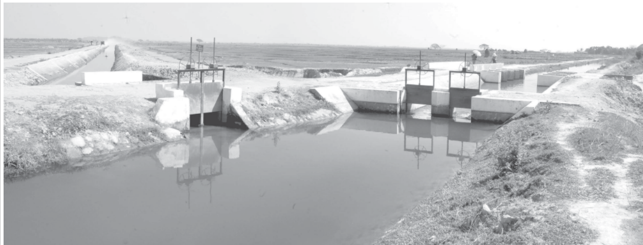
Mouths of left and right canals of Pyaingchaung Dam in Kyauktaw Township.
