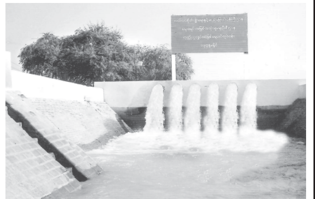
Kokkohla river water pumping station pumping water from Ayeyawady River to be supplied to 5,000 acres of arable land near Kokkohla Village of Pakokku District.
