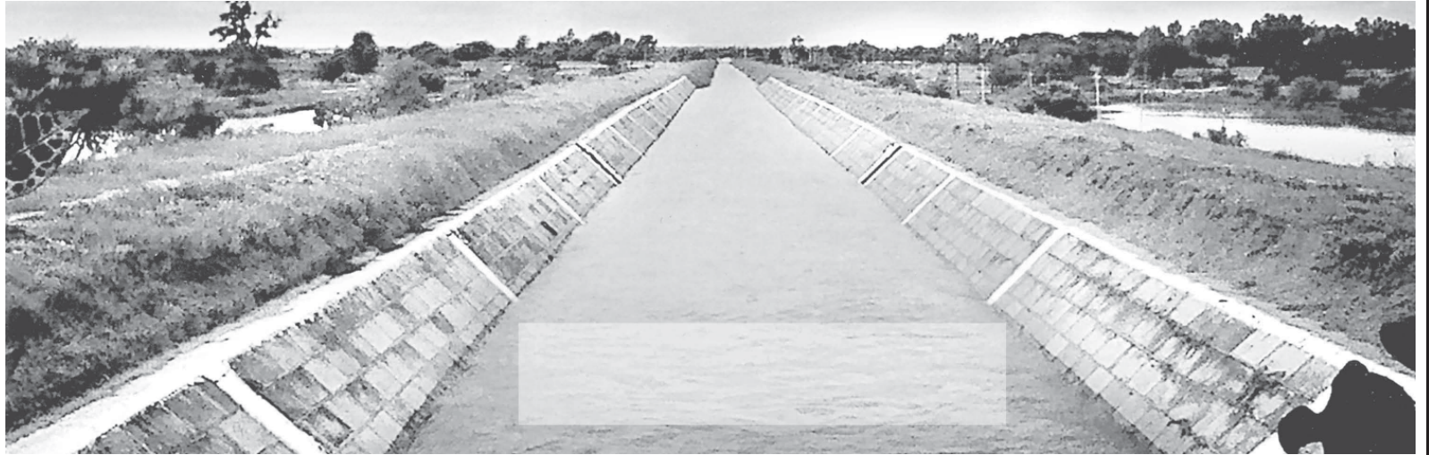
60,000-foot main canal of Kokkohla pumping station supplying water to 5,000 acres of farmland.
