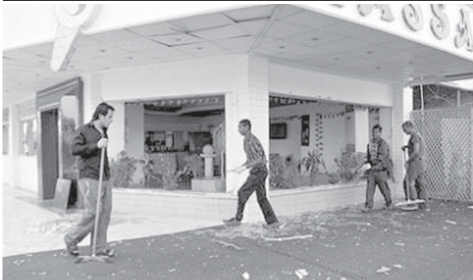
Shattered glass is cleared away at a popular restaurant damaged following a road side bomb that detonated along a popular street in central Baghdad.— INTERNET
