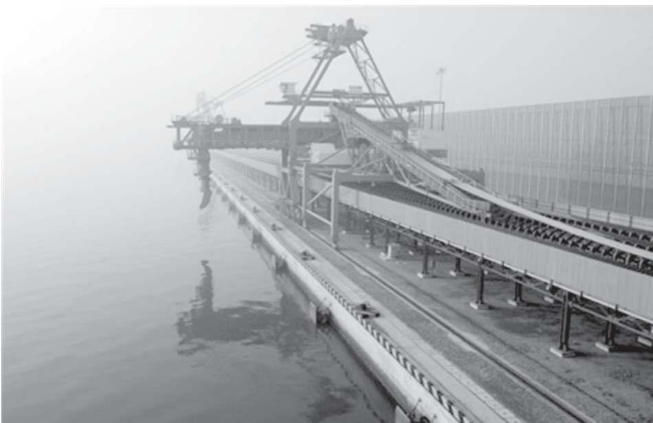
Photo taken on 2 March, 2009, shows the coal dock of the Caofeidian industrial zone in Tangshan, north China's Hebei Province. Caofeidian, an island-turned 50-sq km development zone in the Bohai Bay, has developed a port handling capacity of 100 million tons per year, with the establishment of an ore dock, a crude oil dock and a coal dock.—XINHUA
