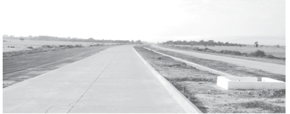
Photo shows already-built Myochaung-Thagara road section at mile post (146/0). —MNA
