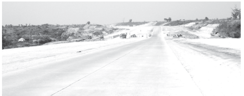
Photo shows already-built Myochaung-Thagara road section at mile post (119/0). —MNA
