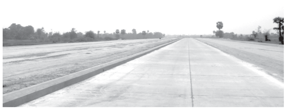
Photo shows already-built Myochaung-Thagara road section at mile post (142/6). —MNA
