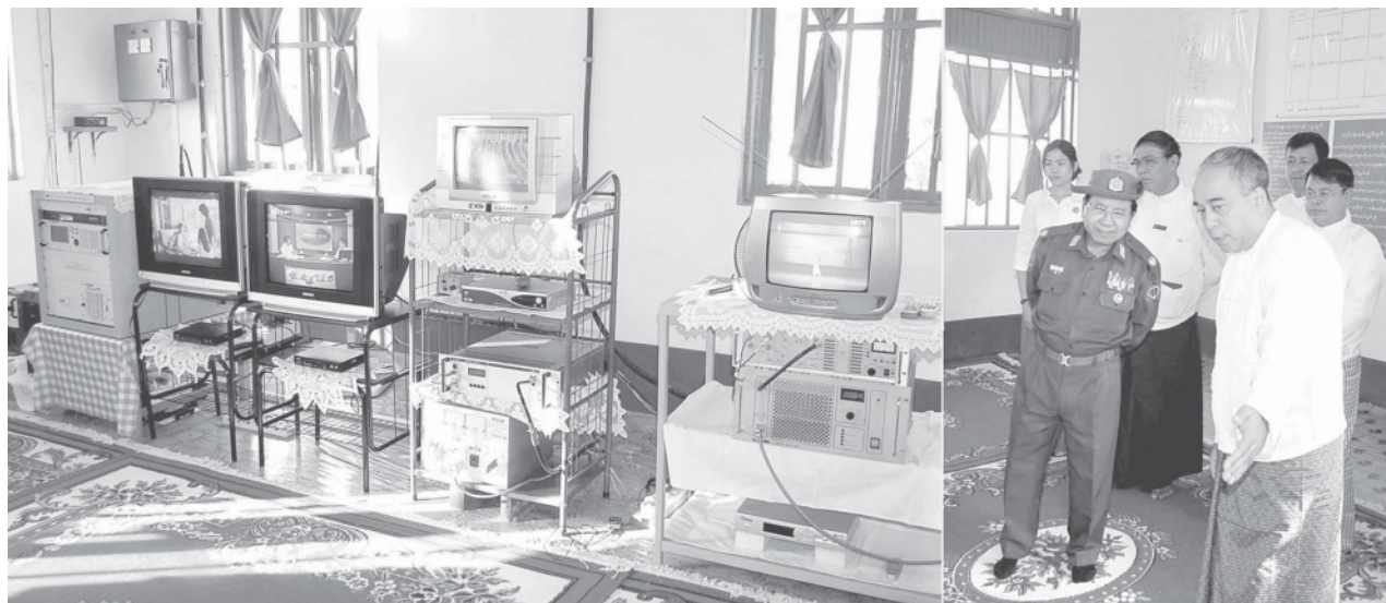
Minister for Information Brig-Gen Kyaw Hsan inspects broadcasting of MRTV-4 and related TV channels at Myanma Radio and Television Retransmission Station in Thandwe.—MNA
