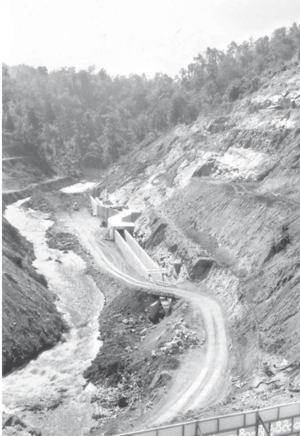
Diversion conduit seen near Nancho Creek.
