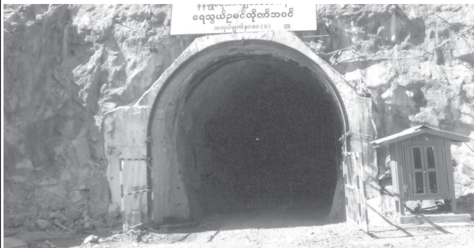
Photo shows entrance to intake tunnel of Nancho Hydropower Plant.
