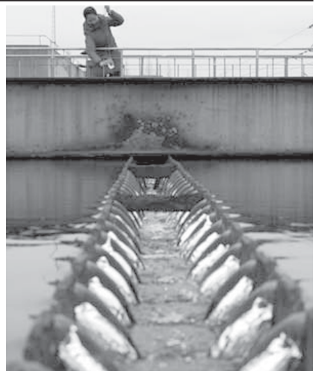
A woman worker takes a glass of water for tests from the filter pool after the contaminated water plant resumed operations in west Yancheng City, east China's Jiangsu Province, on 23 Feb, 2009.—XINHUA
