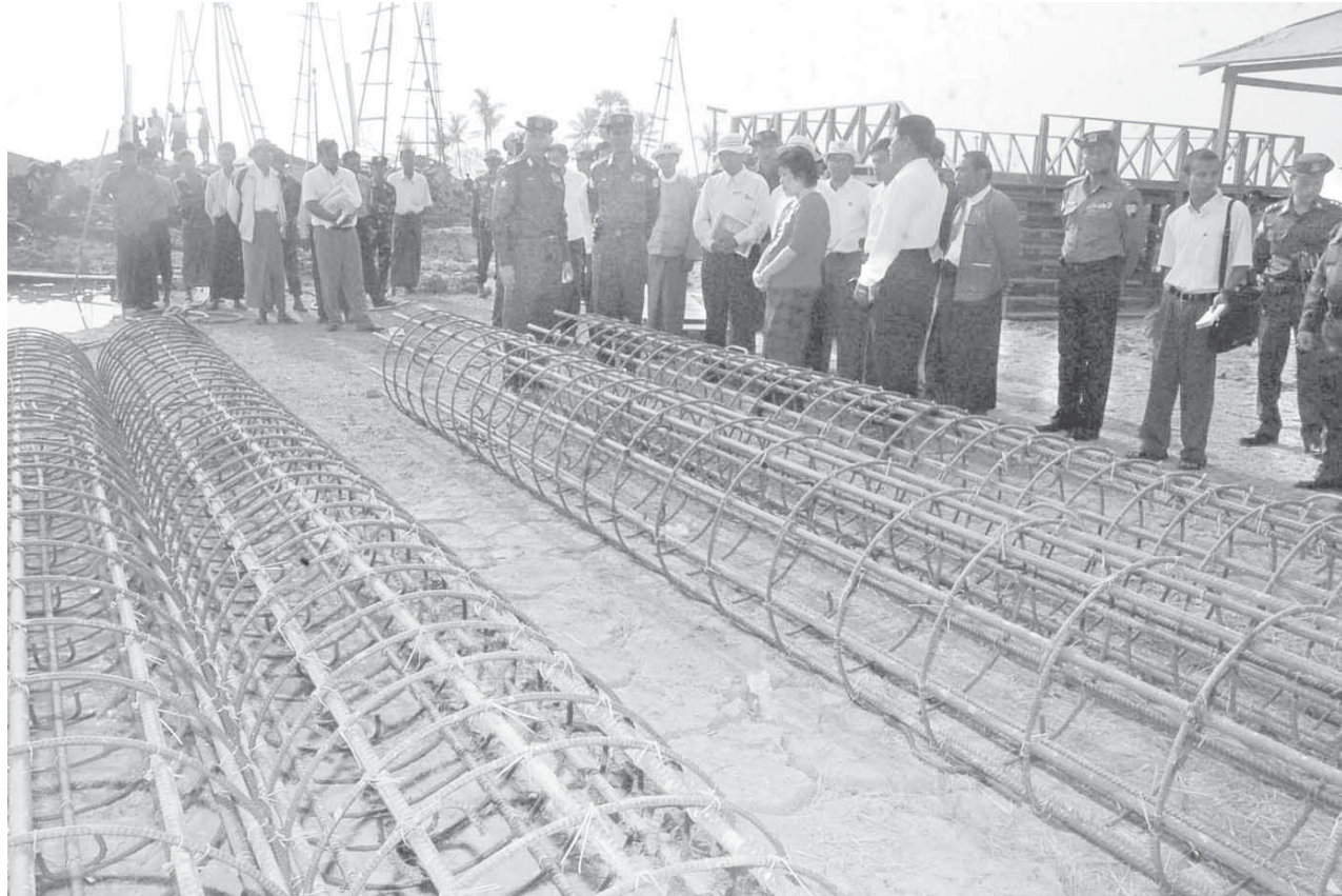
Maj-Gen Ko Ko of Ministry of Defence inspects construction of cyclone shelter at Daminseik village in Pyapon Township.—MNA
