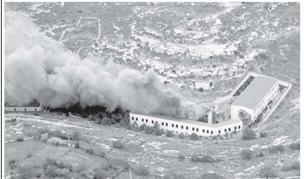
An aerial view shows an immigration centre burning on the Mediterranean island of Lampedusa on 18 Feb, 2009. Fourteen people were being treated for smoke inhalation but no one was seriously injured, Italian media reported.
