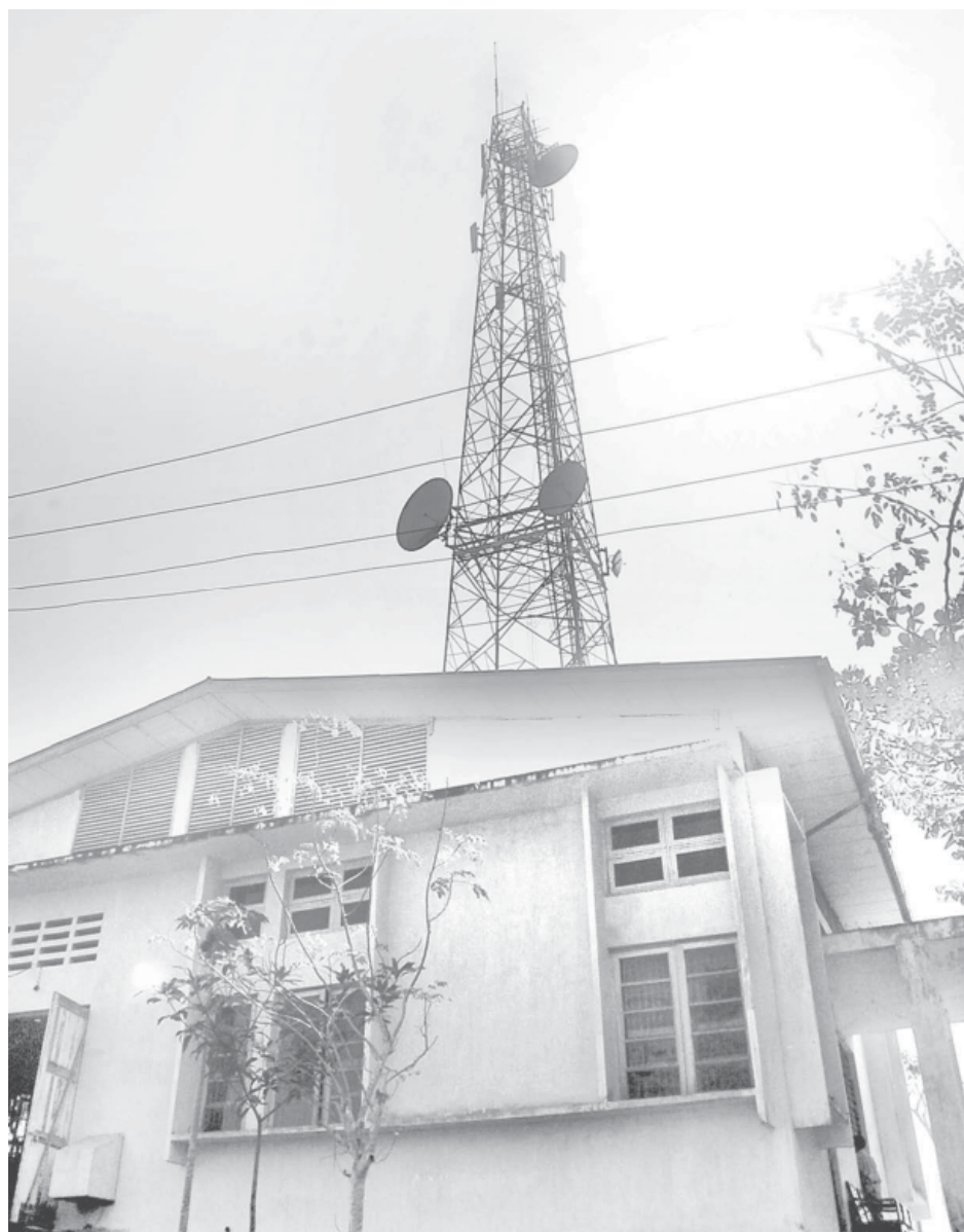
A station indicates improvement of communication sector in Mon State.
