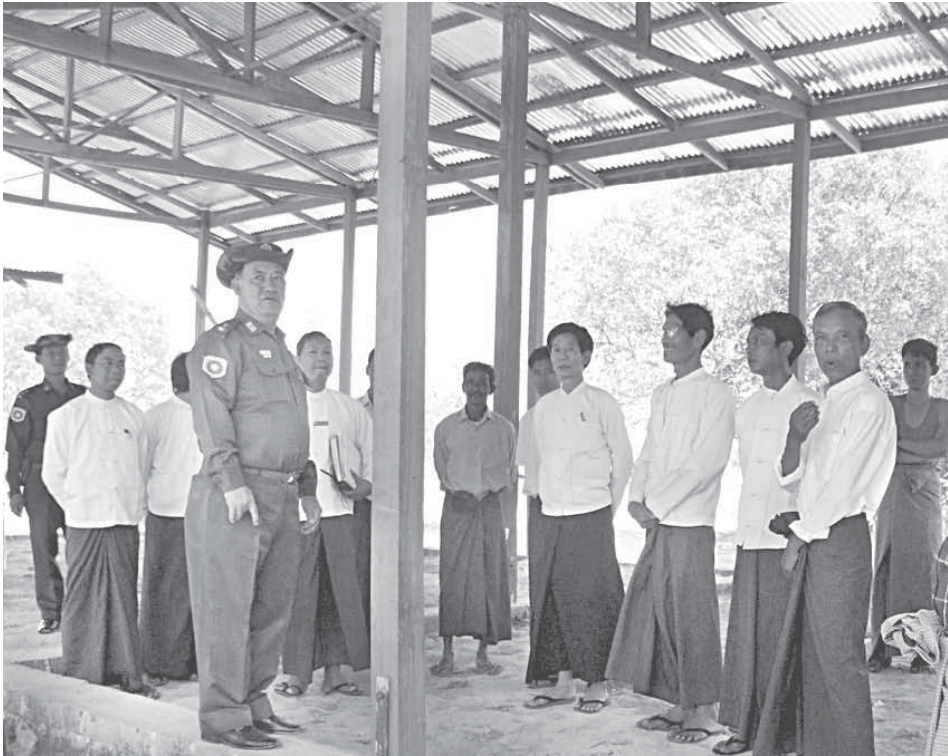
Minister for Home Affairs Maj-Gen Maung Oo inspects the construction of the new school building in Nyaunglunt village BEMS.—MNA
