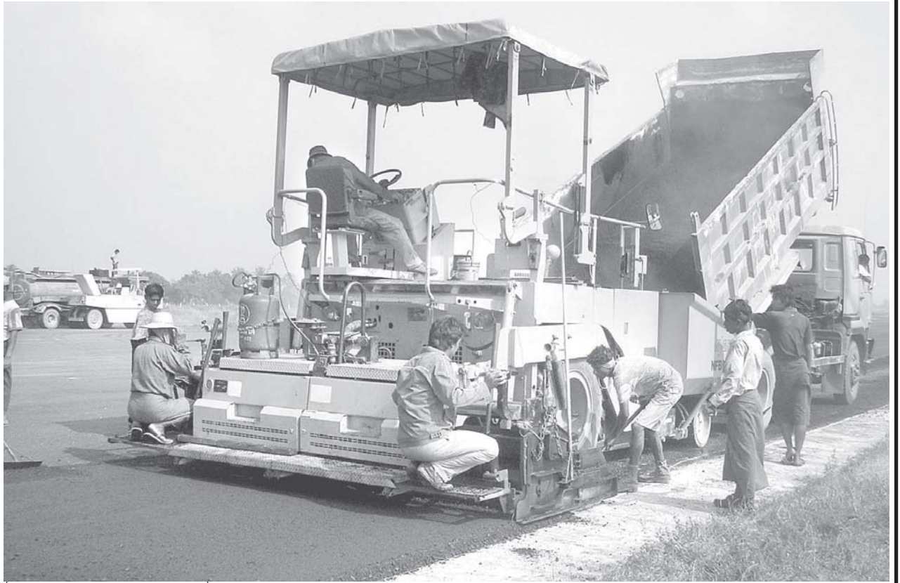
Workers resurfacing the runway.
