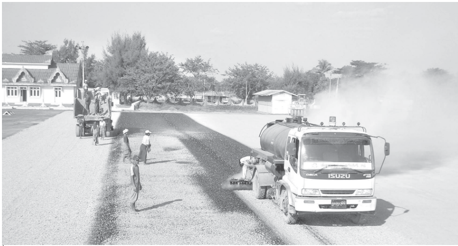
The tarring of the runway in progress.
