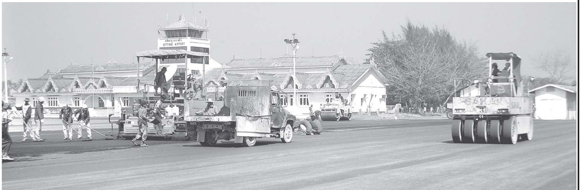
Road rollers at work to resurface the apron.
