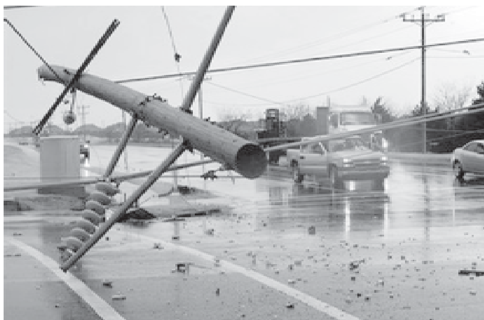
Utility poles block part of an intersection after they were blown over in Oklahoma City, on 10 Feb, 2009. A series of storms, with at least one tornado reported, swept through central Oklahoma on Tuesday afternoon.—INTERNET
