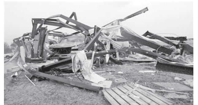
A building containing the business of Four Seasons Paintless Dent Removal is shown after winds from a tornado knocked down power lines, damaged homes and businesses on 10 Feb, 2009, in Edmond, Okla.—INTERNET
