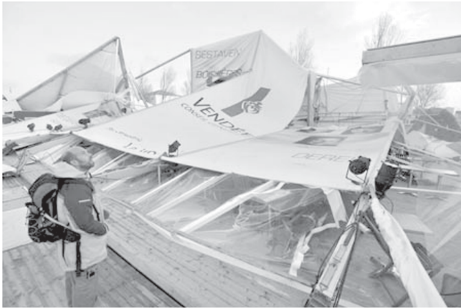
A man watches fallen temporary house hit by high winds in Les Sables d'Olonne, western France, on 10 Feb, 2009. High winds lashed France on Tuesday, prompting authorities to shut Paris' three international airports.—XINHUA
