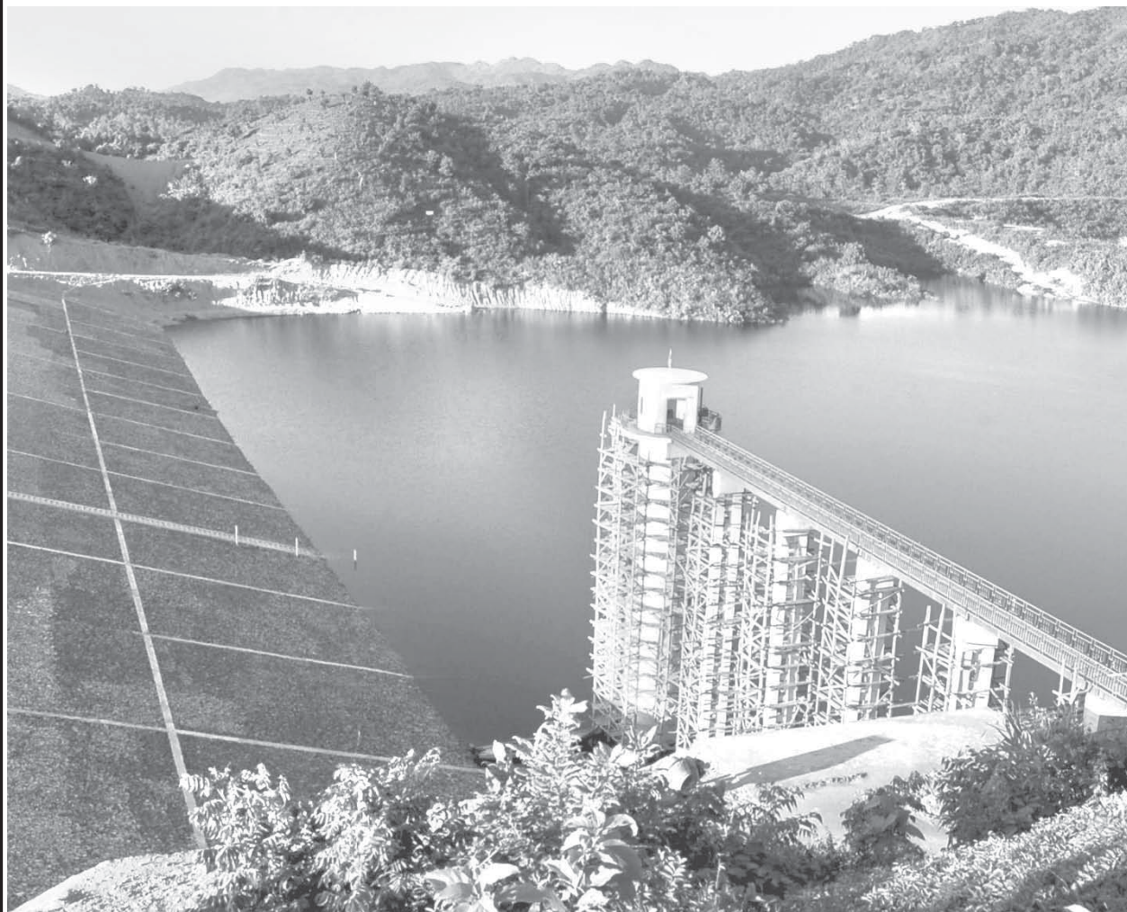
Zichaung Dam in Kyauktaw Township. — MNA
