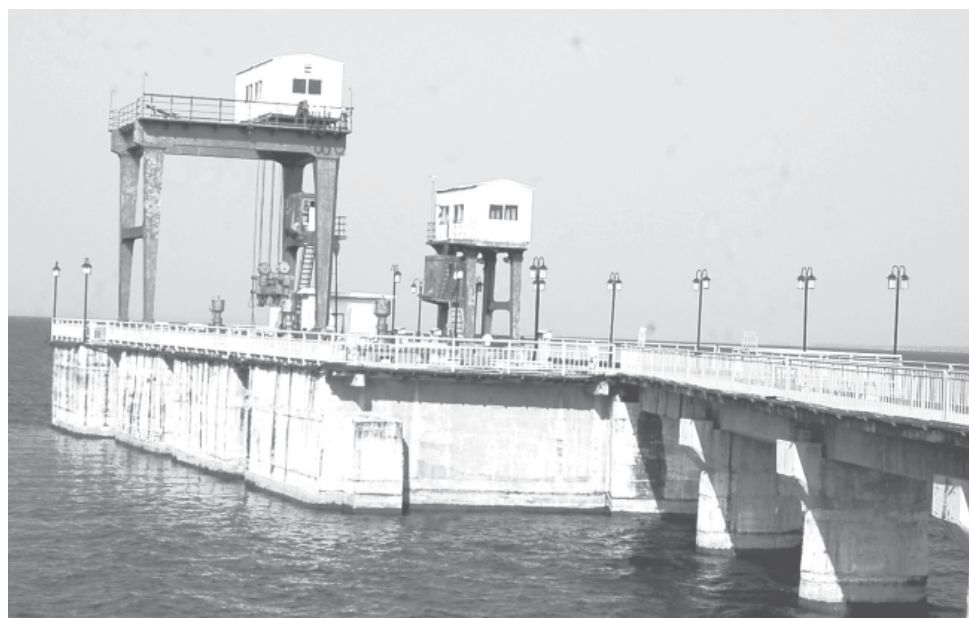
Vice-Senior General Maung Aye inspects Thaphanseik Dam. —MNA
