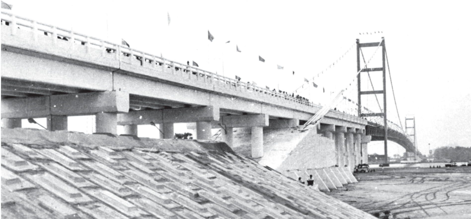
Gyine (Zathapyin) bridge over Gyine River constructed in Kayin State for smooth transportation and speedy flow of goods.
