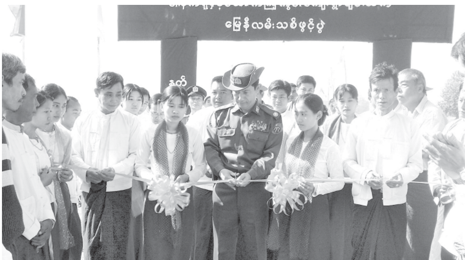
Deputy Minister Brig-Gen Than Htay cuts ribbon to open earth road linking Wanetyon Village and Htaukkyantkwin Village in Nattalin Township.—MNA
