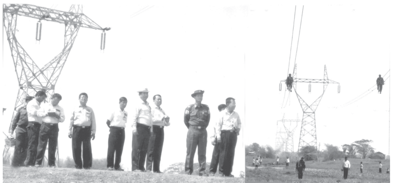
Minister Maj-Gen Khin Maung Myint inspects construction of Kamanat-Thanyin power grid. — MNA
