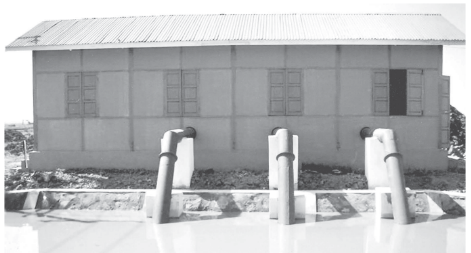
Sitpin river-water pumping station in Hlegu Township.
