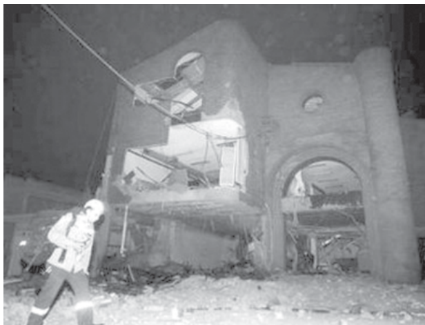
A rescue worker walks in front of a police station after an explosion in Cali on 1 Feb, 2009. A bomb exploded outside a police building in the Colombian city of Cali on Sunday, wounding at least four people in a rare urban attack, officials said.
