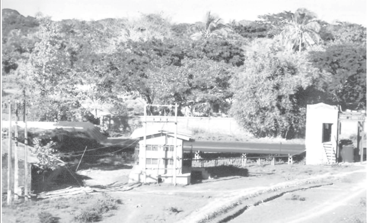
Kyokon river-water pumping station in Htantabin Township. (See page 7)
