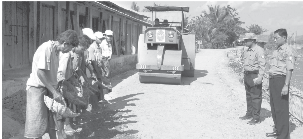
A gravel road under construction in urban area of Buthidaung.
