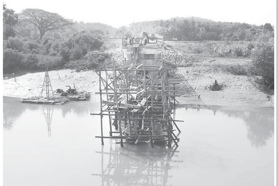
Photo shows 60 per cent completion of building Karuppi Creek Bridge.
