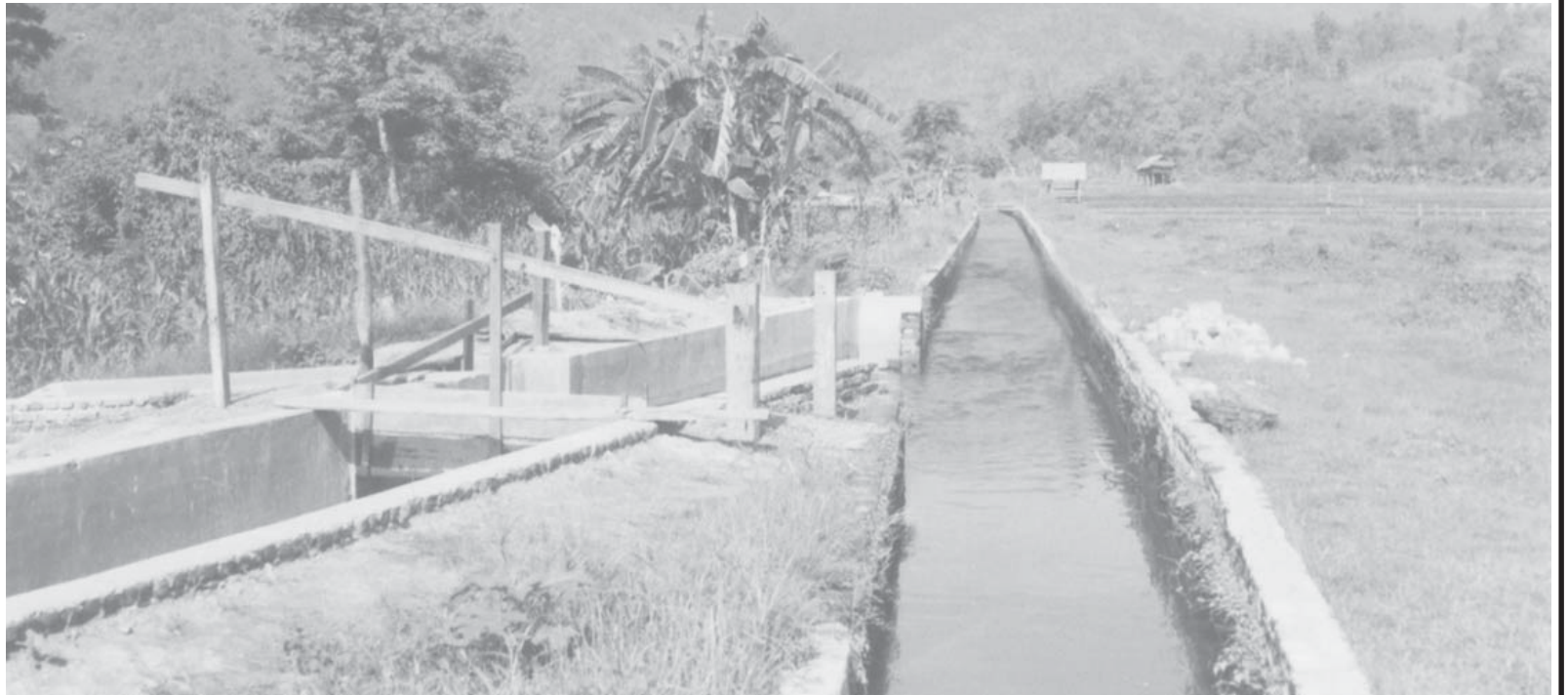
The six-foot-wide and 200-foot-long canal, through which the water of Nanpalaw Creek in Tiddim Township is drained to generate hydroelectricity.
