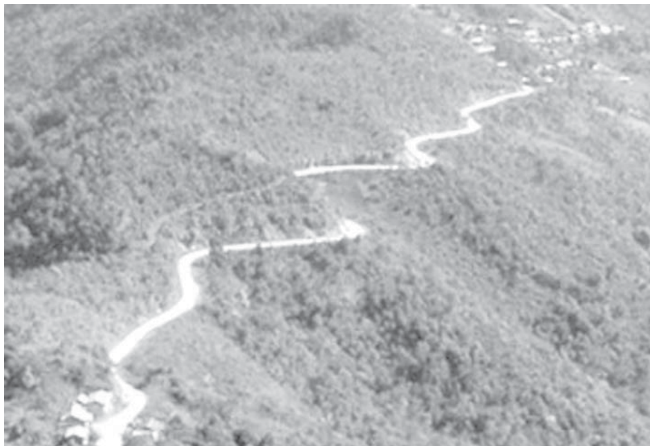
An aerial view of Kalay-Tamu Road.
