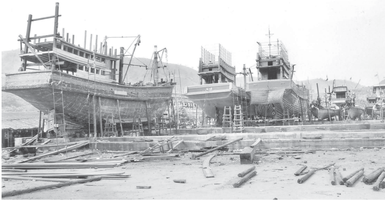
Ships and trawlers in dock for repairs and being built in the dry dock of Thida Dry Dock in Kawthoung.
