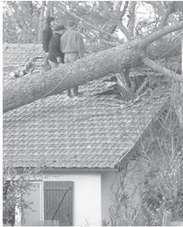
Men work on top of a tiled-roof house to remove branches from an uprooted tree after a winter storm with high winds hit Lege Cap-Ferret in southwestern France on 24 Jan, 2009.—INTERNET
