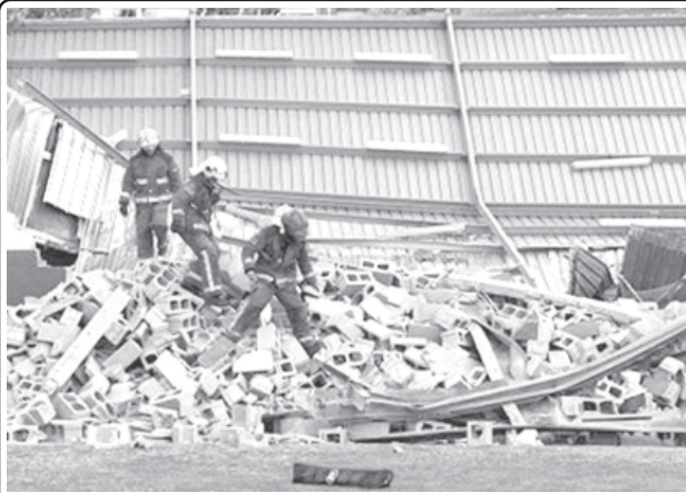
Emergency services work at a sports hall where high winds brought down part of a wall killing four children near Barcelona. Hurricane-force winds lashed Spain and France Saturday, killing at least 14 including four children when part of a sports hall collapsed, while nearly two million were left without power.—INTERNET
