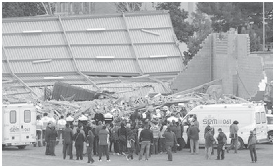
Rescuers work in part of a sports center which collapsed in high winds killing four children and trapping and injuring others in Sant Boi de Llobregat, Spain, on 24 Jan, 2009. Freak weather conditions have caused winds gusting to 160 kph (100 mph) in many places throughout Spain. A woman died when a wall fell on her in Barcelona and a traffic officer was killed by a falling tree in northwest Galicia.—INTERNET
