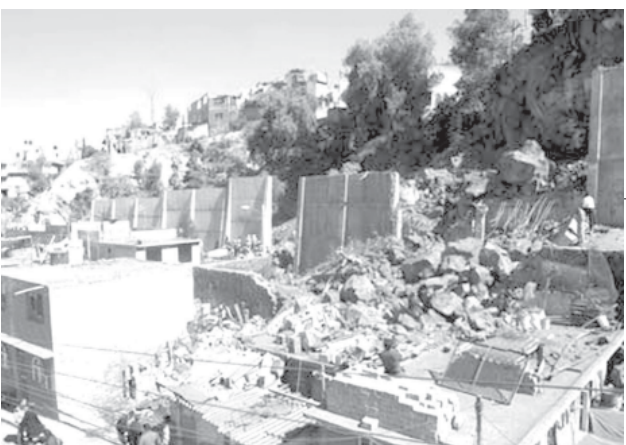
Photo taken on 22 Jan, 2009 shows a scene of a landslide in Mexico City, capital of Mexico, on 22 Jan, 2009. The landslide caused two people dead with another one injured. The reason is estimated to be the loose structure of the hill caused by continuous heavy rains last year.— INTERNET
