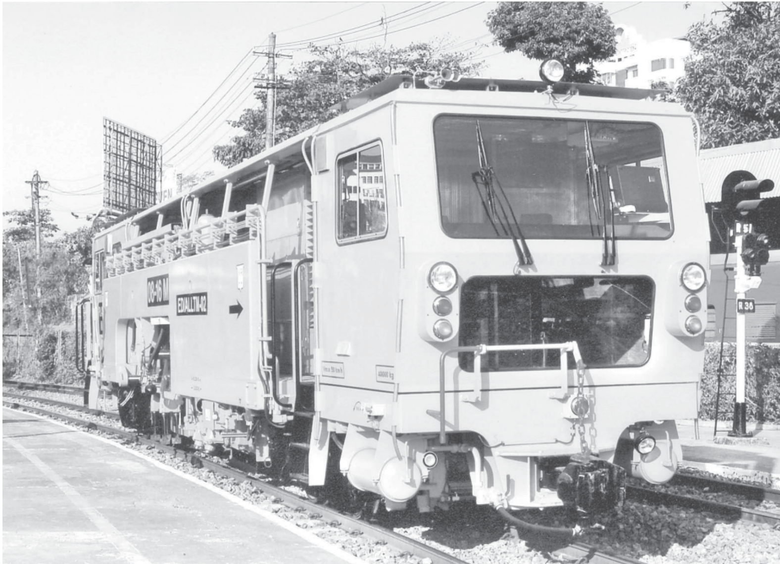
The automatic levelling, lining & tamping machine imported from India.
