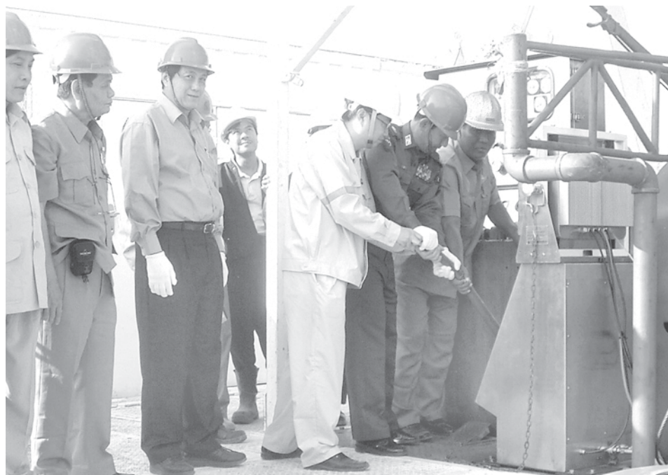
Deputy Minister for Energy Brig-Gen Than Htay and foreign technician Mr. Zhang Yingzh start operating the machine to sink Shwe Pin Test Well No. 1 in Maubin.—MNA
