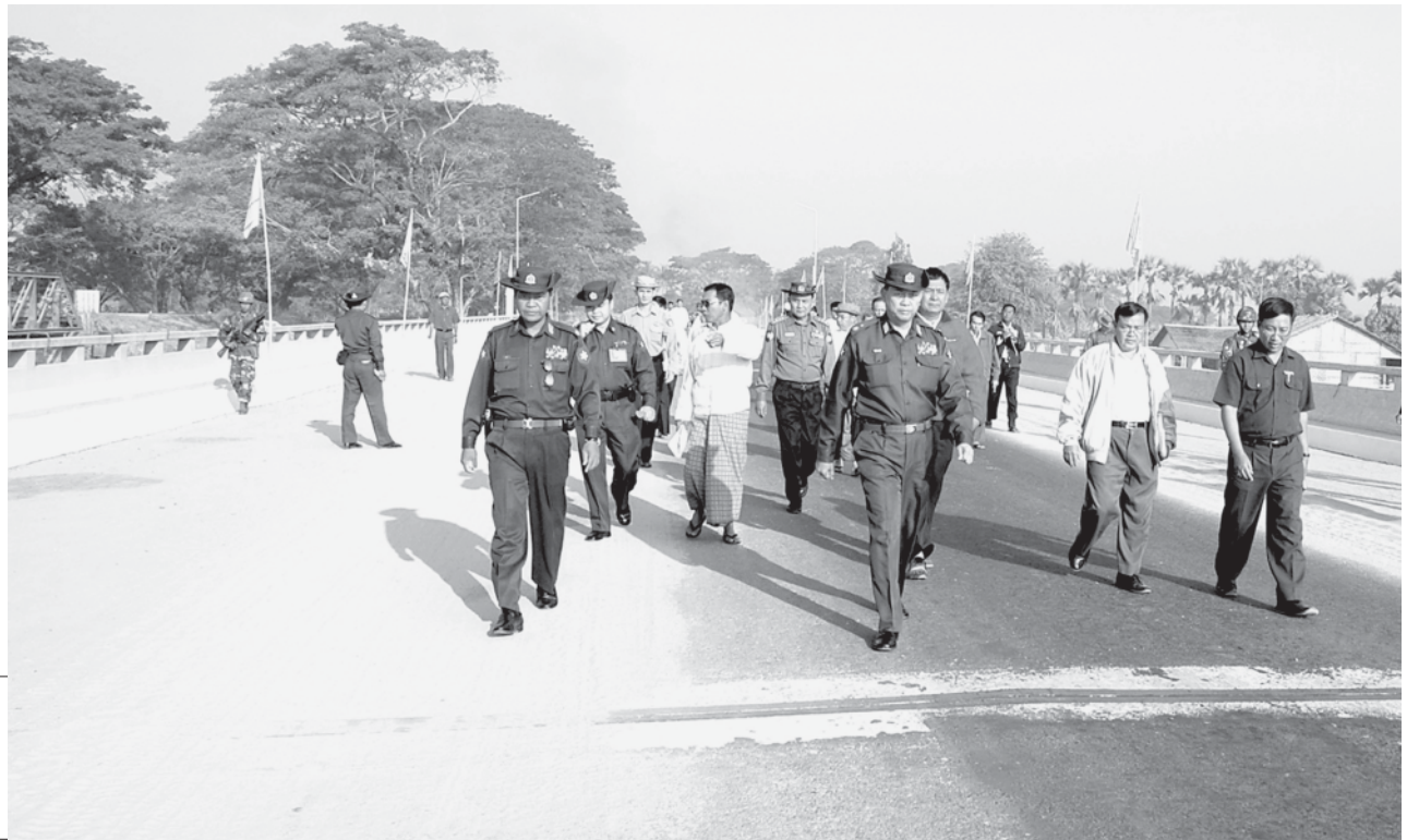
Maj-Gen Ko Ko of the Ministry of Defence inspects Swa Creek Bridge in Yedashe Township, Bago Division.—MNA
