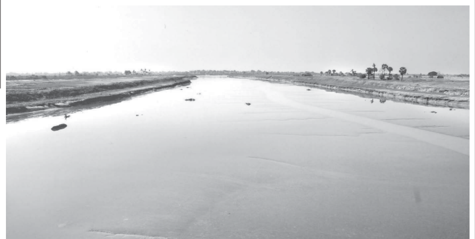
Photo shows silted area and sea water that cannot flow into Yinnye in Creek due to blockage of Yinnye in Sluice Gate.
