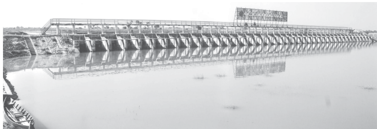
Yinnye in Sluice Gate built with 40 valves in Kyonhtaw Village of Paung Township to control the inflow of sea water and supply of fresh water.
