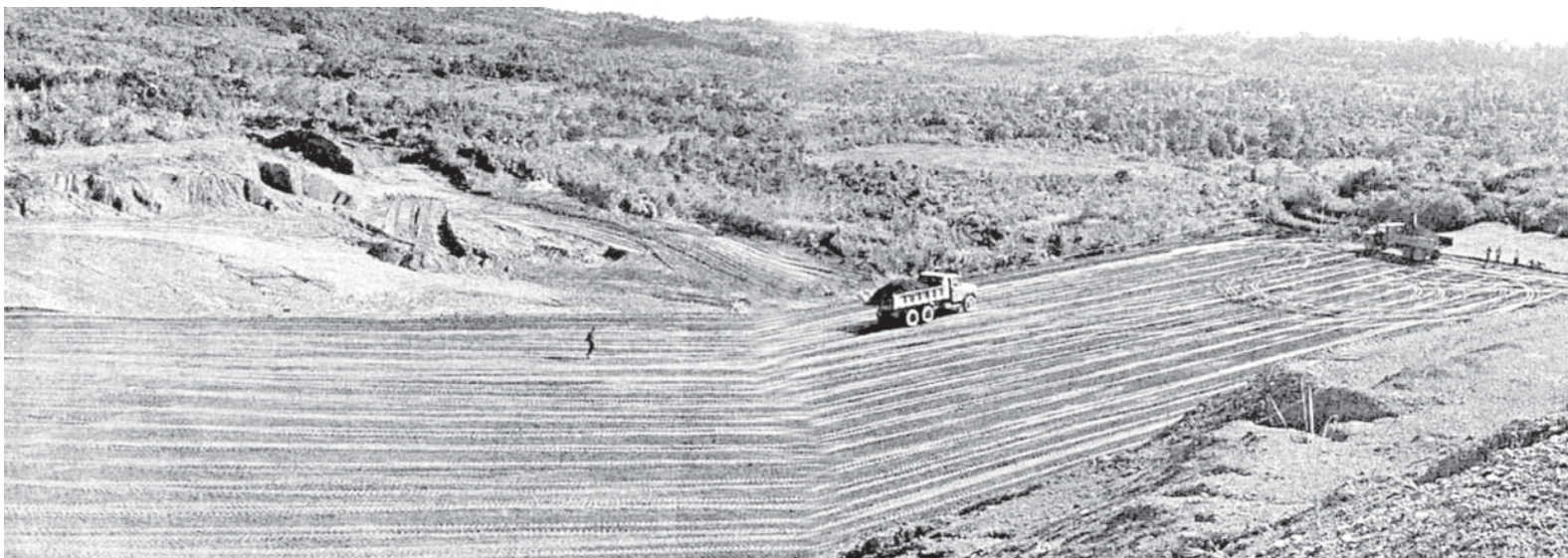
An aerial view of the construction site.
