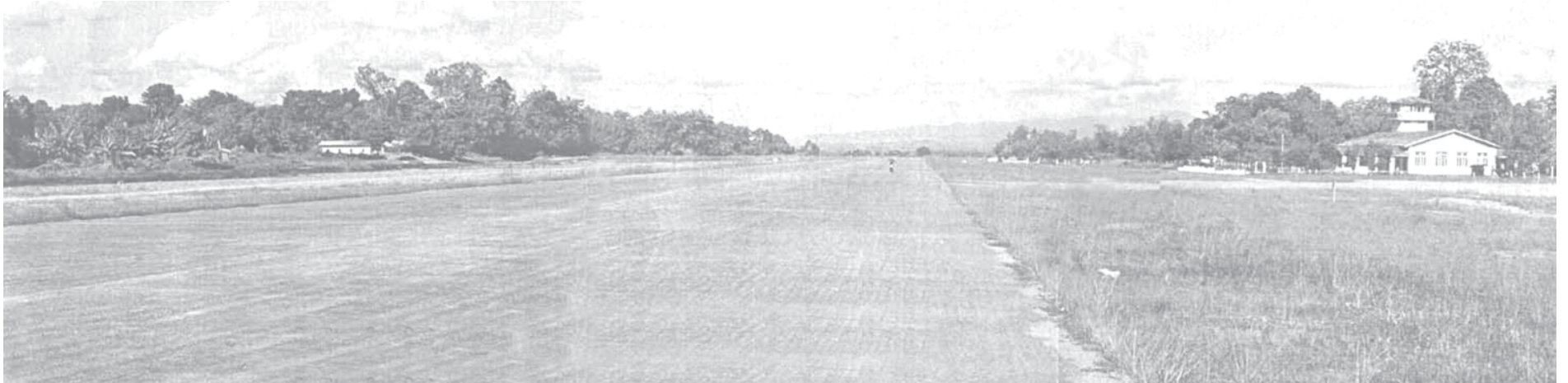
The runway of Khamti Airport being upgraded to a fine one.
