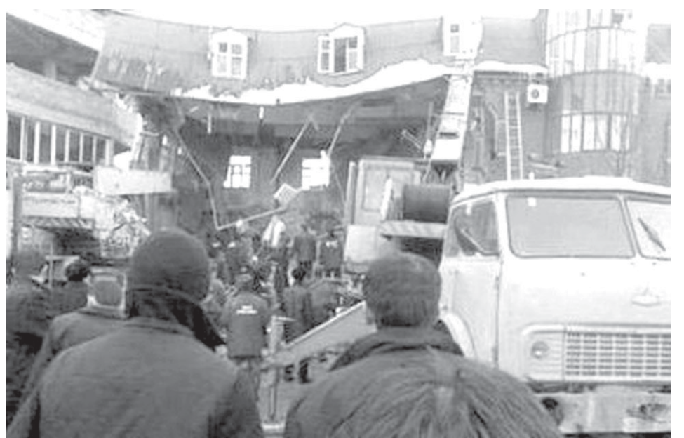
People stand in front of a building destroyed by a blast in Russia's southern city of Nazran, on 13 January, 2009. The explosion in the region of Ingushetia in southern Russia destroyed a government office on Tuesday and buried people underneath rubble. The cause of the blast was unclear, but Itar-TASS news agency quoted the speaker of Ingushetia's parliament as saying that a gas leak may have caused the blast.—INTERNET
