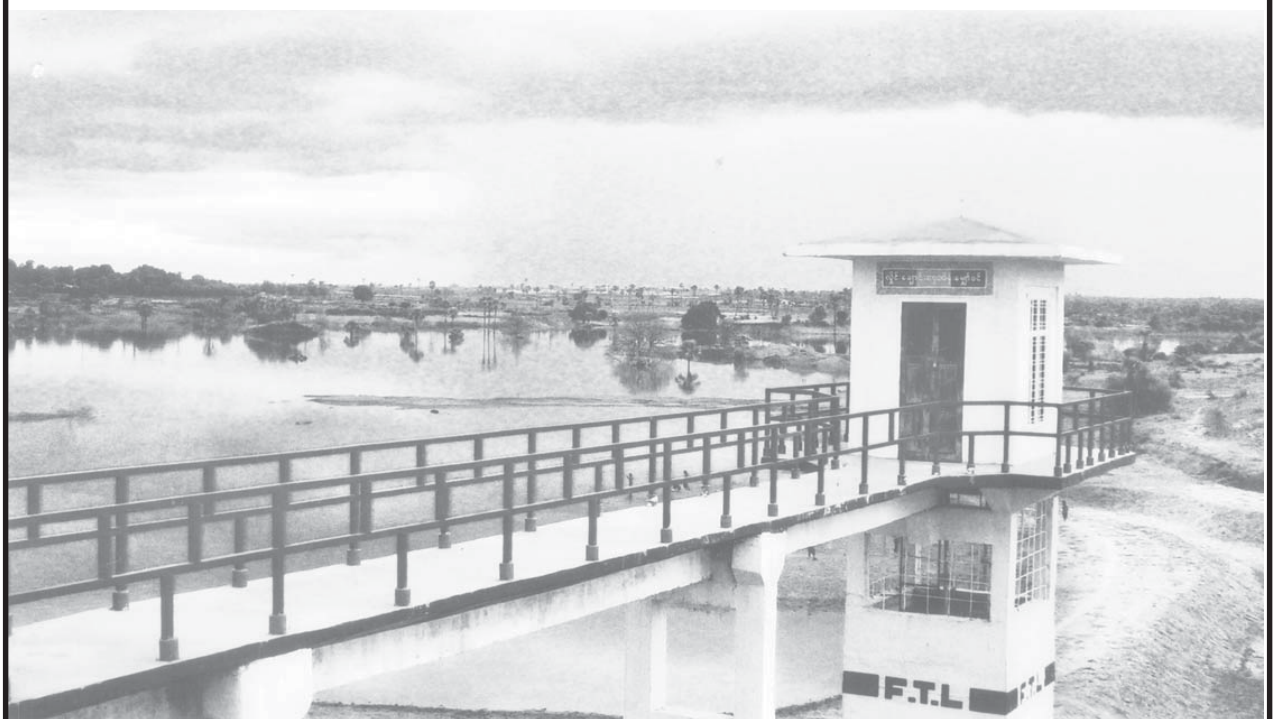
Control tower of Hlaingchaung Dam near Nwe-in Village, Pale Township, Sagaing Division.
