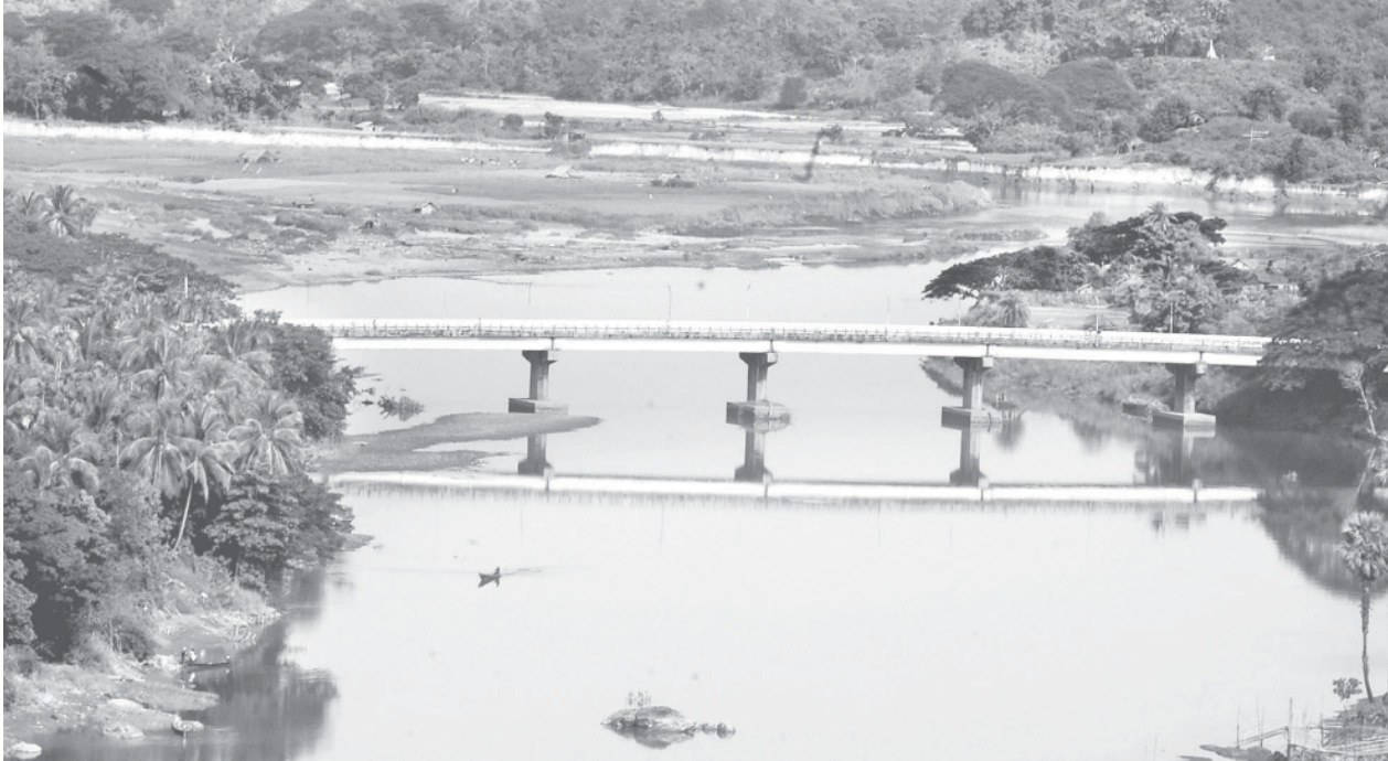
The 540 feet long Dwarawady Bridge linking Taungup and Thandwe.
