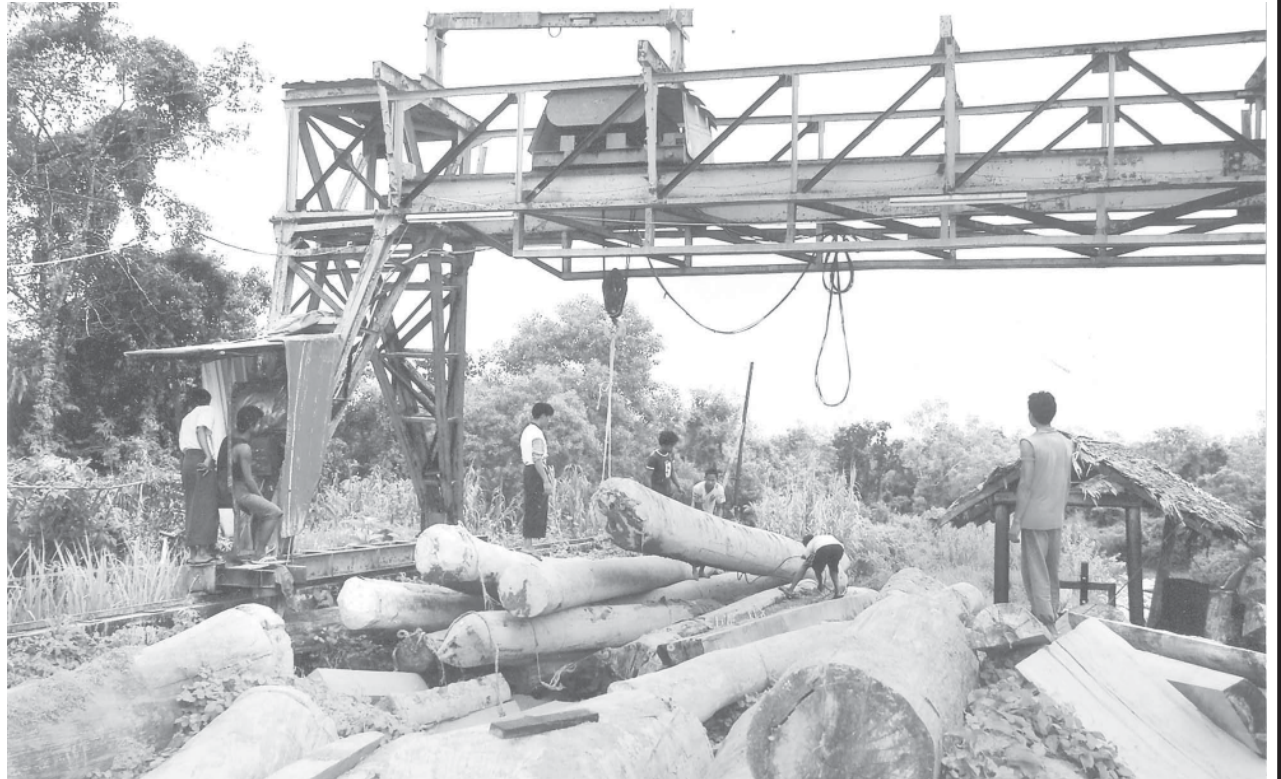
Timber logs being lifted by crane for making plywood.
