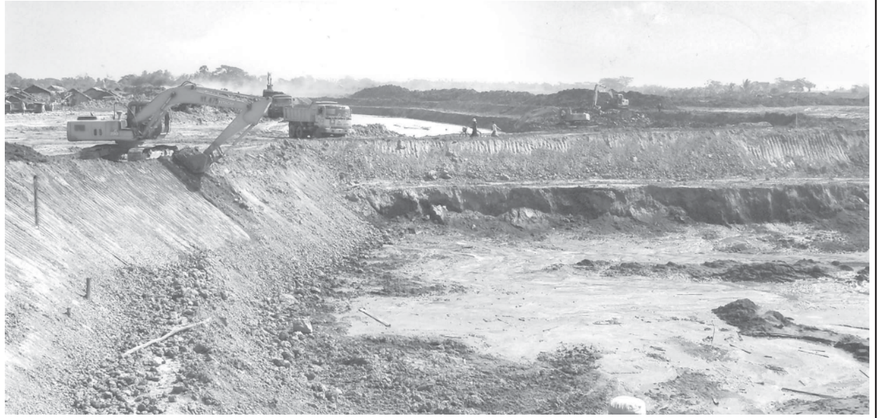
A construction site of Kadappana Sluice Gate Project.
