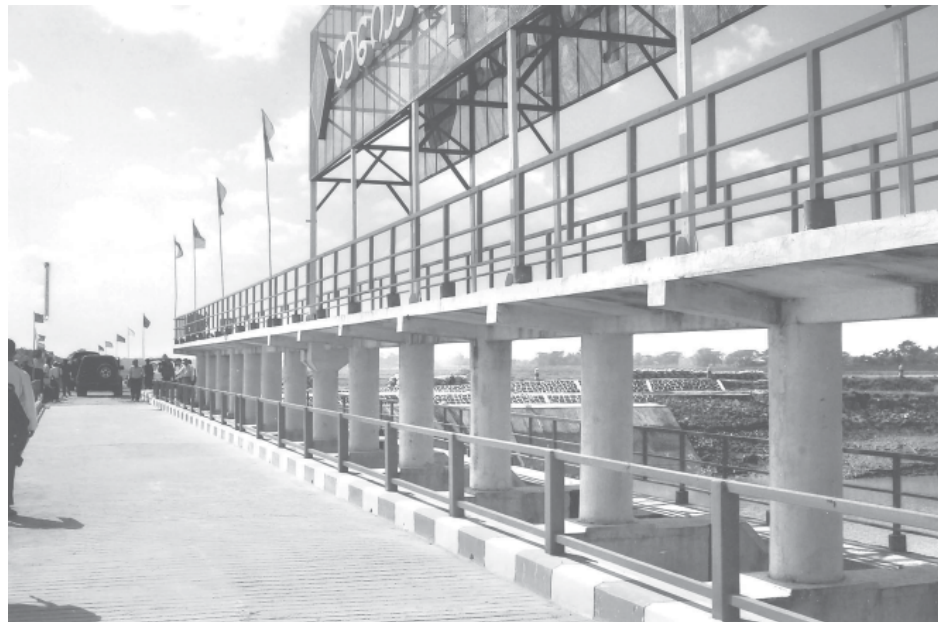
Dagaw Sluice Gate near Dagaw Village in Thongwa Township benefits 15,000 acres of arable lands.
