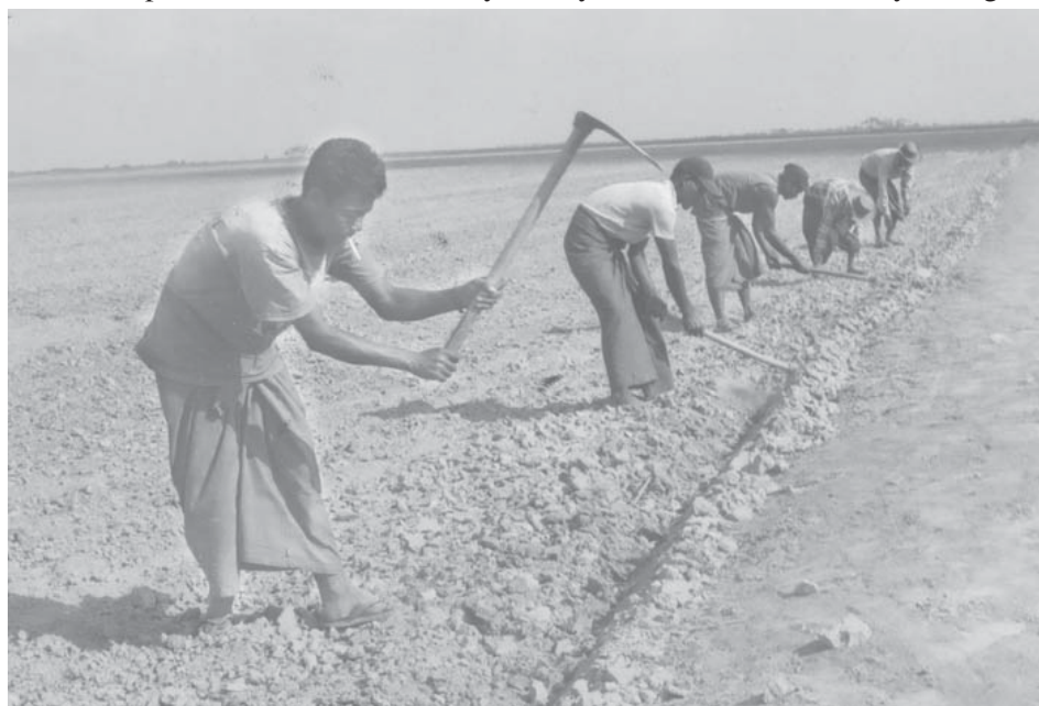
Workers carrying out land preparation work.
