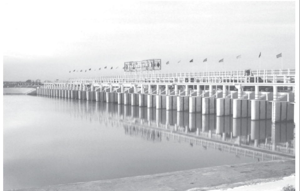
Kayan Sluice Gate near Chaungwa Ywahaung Village in Thanlyin Township on completion will be able to irrigate 30,000 acres of farmlands.
