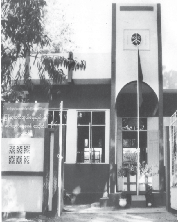
Myanma Posts and Telecommunications Centre constructed in Ahlon of Monywa Township for enhancement of communications sector.
