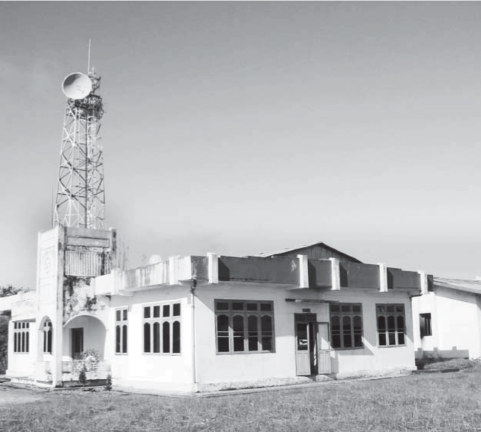
Communication Station built in Falam of Chin State to ensure development of communications sector for all regions of the country including border areas.
