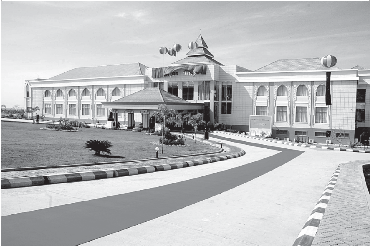
Main Building of Yatanarpon Teleport seen in Yatanarpon Myothit of PyinOoLwin Township.
