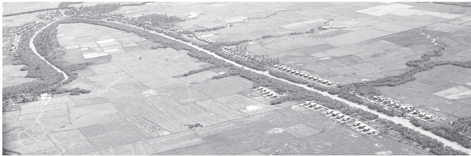
Land allotted for building of houses in Kwinkaut village of Mawlamyinegyun Township.—MNA
