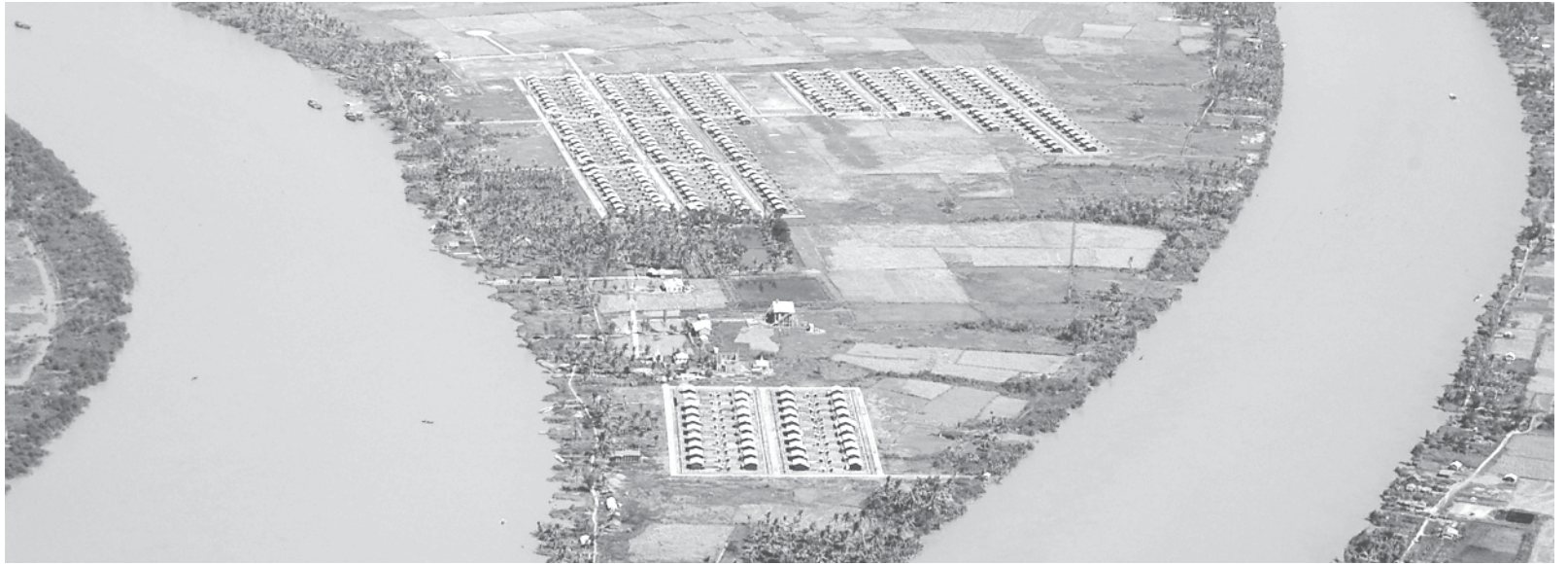
Land allotted for building of houses in Kyatshar village of Mawlamyinegyun Township.—MNA
