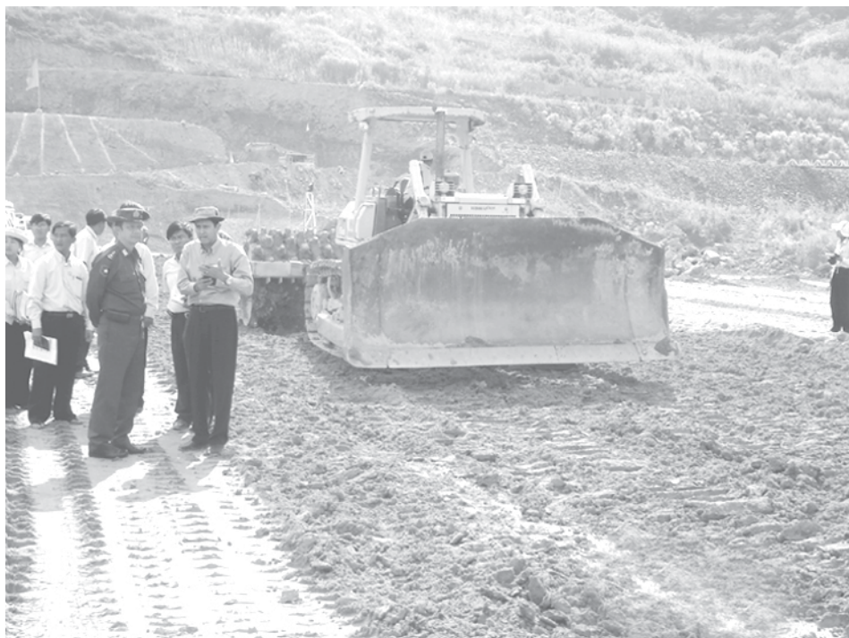
Minister Col Zaw Min inspects Pyu Creek Hydro-power Project.
