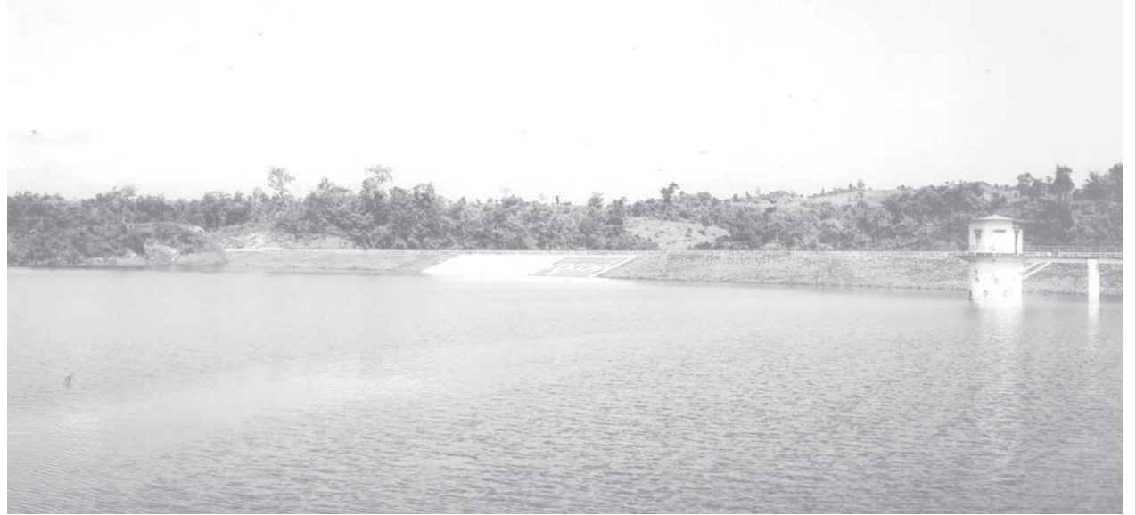
North Yama Supporting Dam storing water to the brim.
