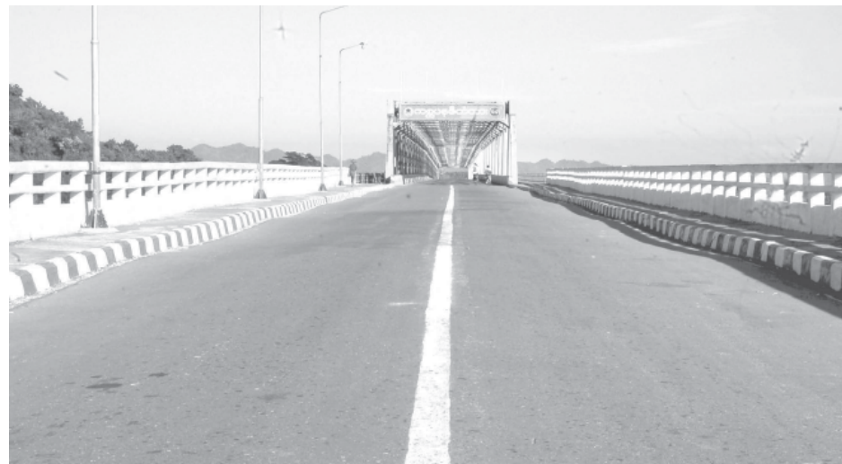
Kissapanadi Bridge in Kyauktaw Township, Rakhine State.
