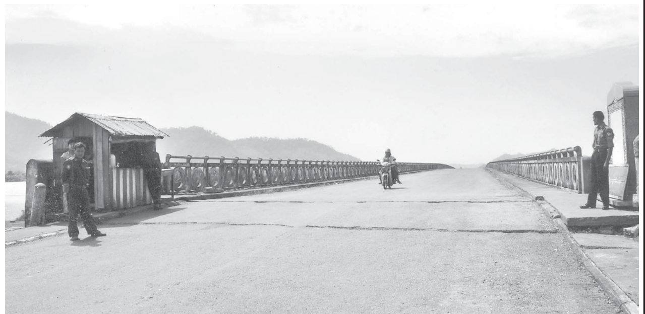
Pathoung Bridge on Myeik-Kawthoung Road spanning the Taninthayi Creek serves as an access to inland areas.
