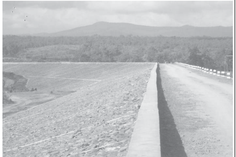
A completed section of the dike of Myittha Multipurpose Dam Project.
