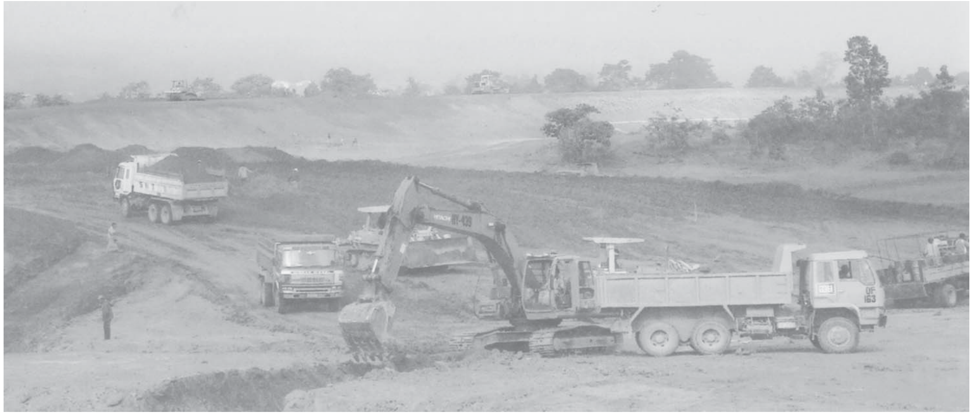
A work site of Myittha Multipurpose Dam Project.
