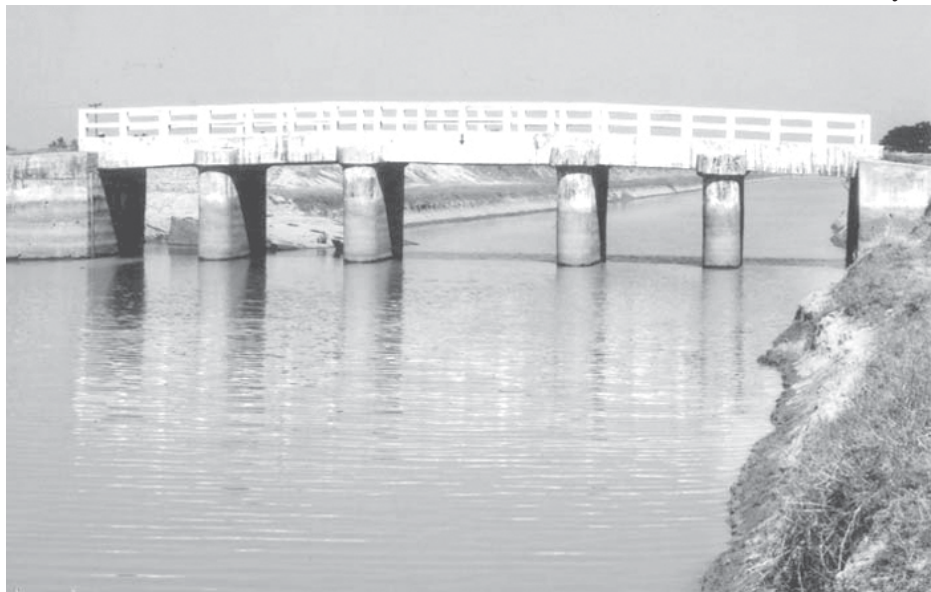
A canal bridge for smooth transport.
