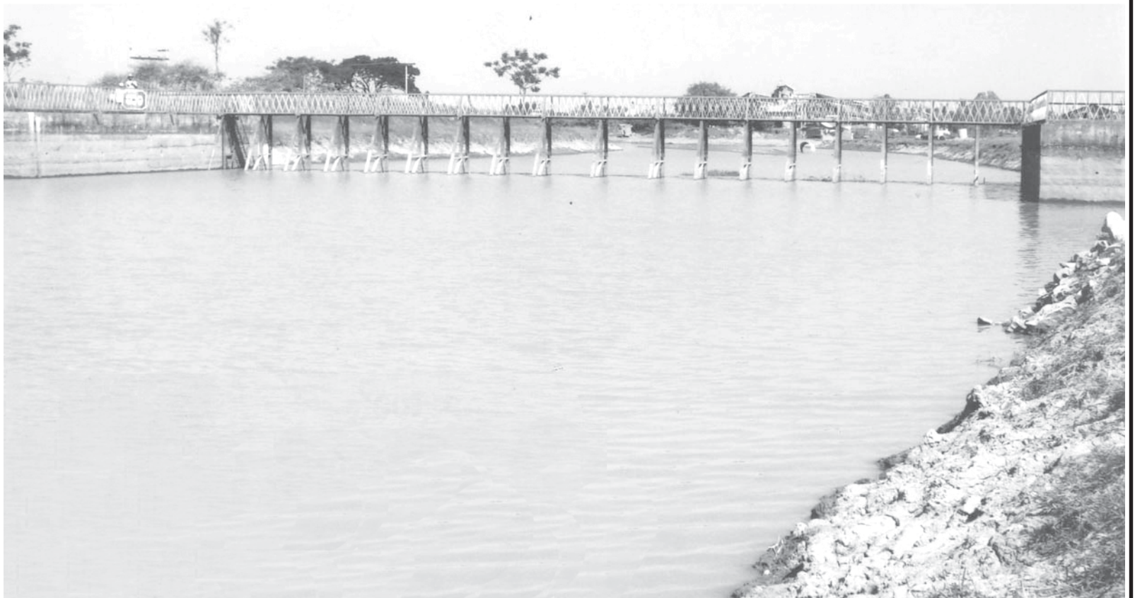
A structure constructed by Construction (6) of Irrigation Department near Ohnhne Village, Thanatpin Township, Bago Division.
