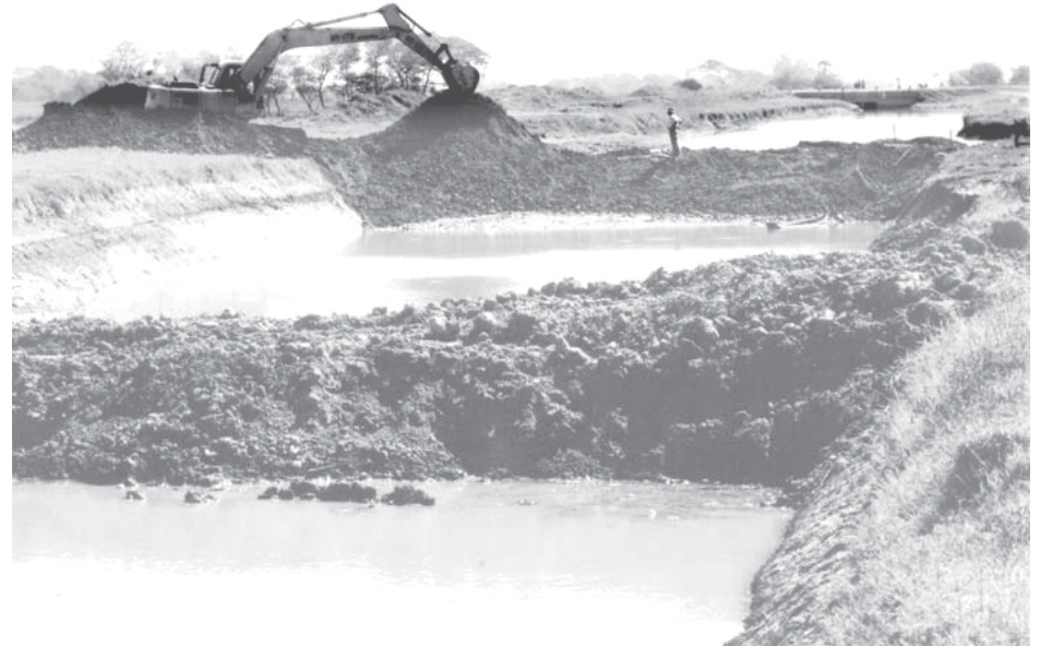
A backhoe at work.
