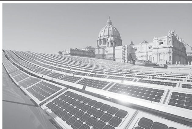
Solar panels are seen on the roof of the Paul VI Hall, at the Vatican. The panels became functional on Wednesday, illuminating and heating Pope Benedict XVI's weekly general audience, held inside the Paul VI Hall.
