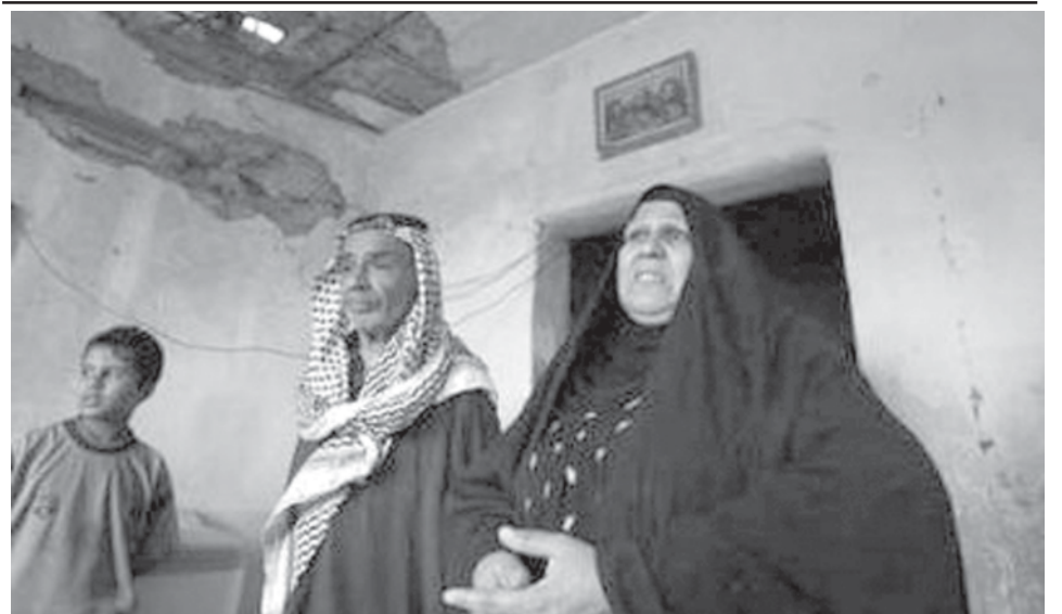
Residents stand under the roof of their house, damaged during fighting in April between the US soldiers and Mehdi army, in Baghdad's Sadr City on 15 Nov, 2008.—INTERNET
