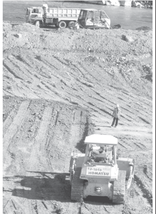
Land consolidation work is being carried out to prevent the stored water from seeping through the dam.
